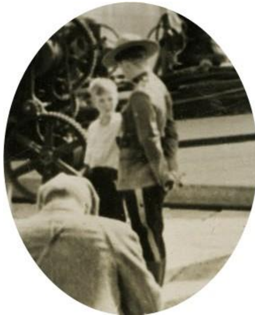
RCMP dockside near SS Tutshi circa 1938 – 1940
