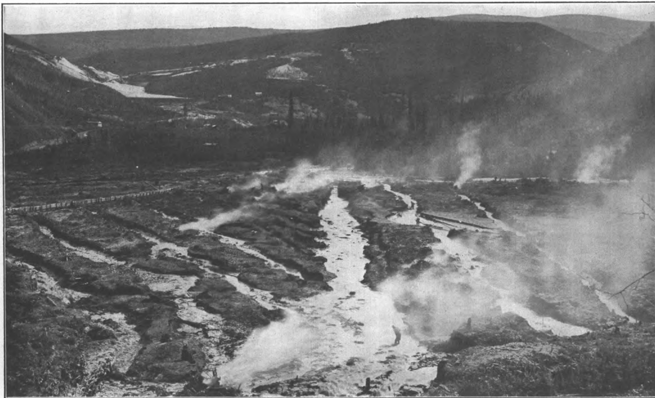
Ground Sluicing.
