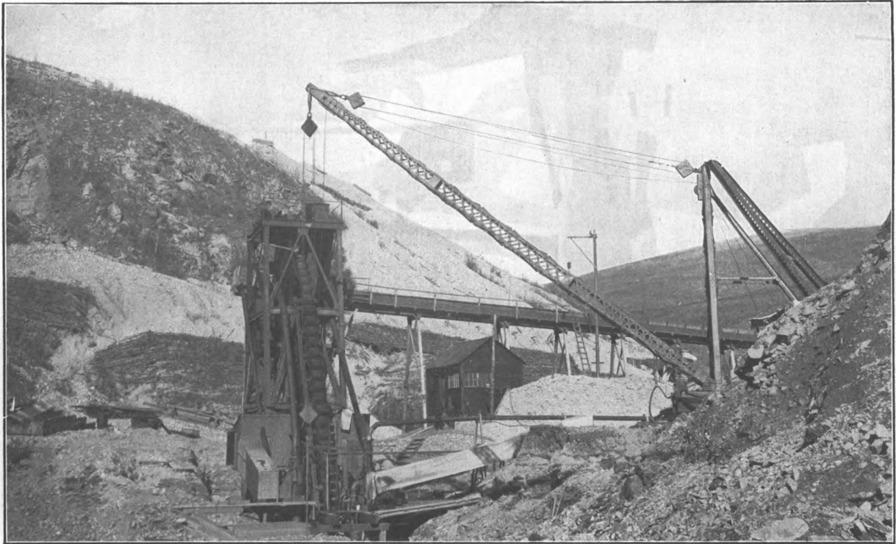
An Electric Hoist on 30 below on Bonanza (Y. C. G. F. Co.)
