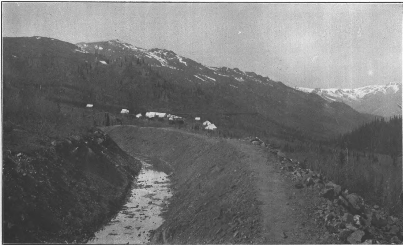
Part of Yukon Gold Co's., water ditch.
