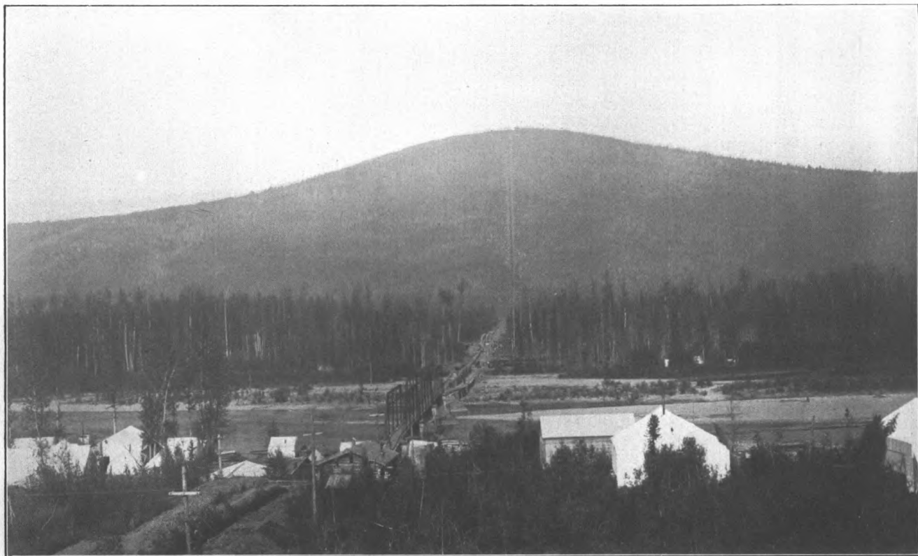
The Y. C. G. F. Co., Pipe Line from Bear Creek.
