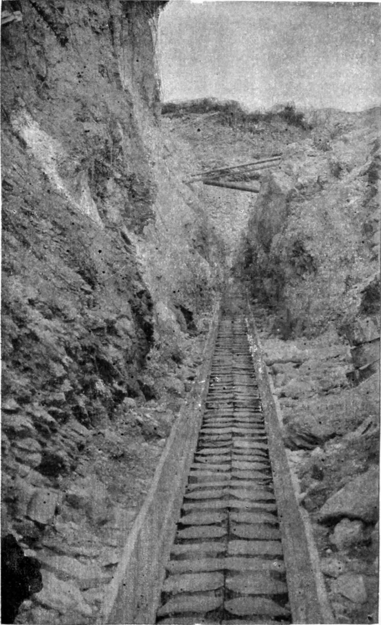
Sluice on Property of J. B. Tyrrell, M. E., Bonanza Creek.
