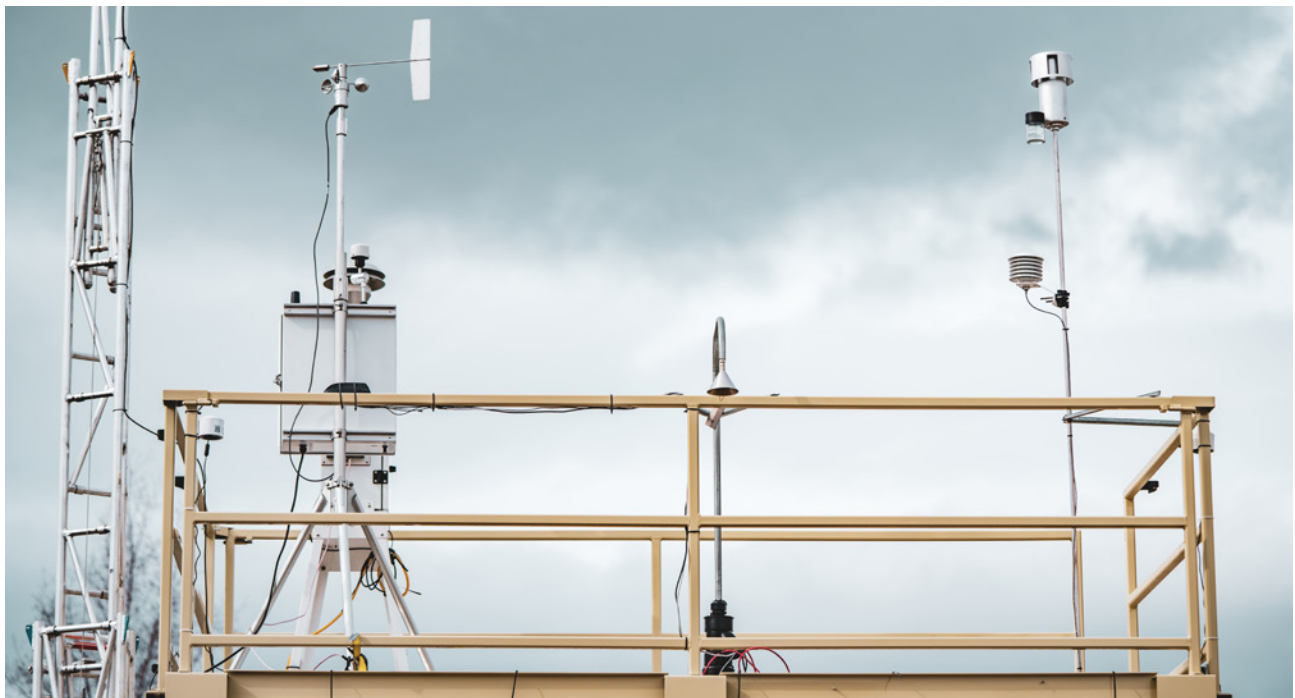
Roof of NAPS station showing sampling equipment.
