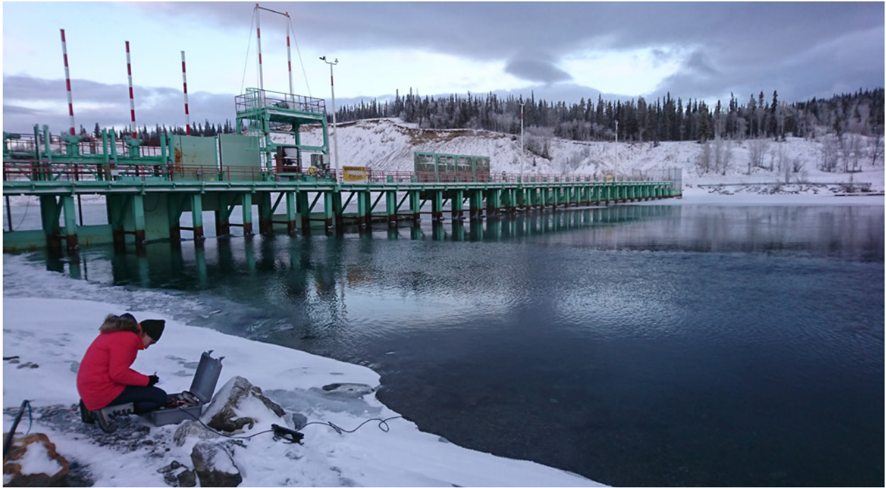
Water quality sampling, Yukon River at Marsh Lake Bridge.
