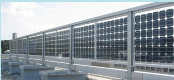
Bifacial (two-sided) solar panels mean more electricity from less space.
