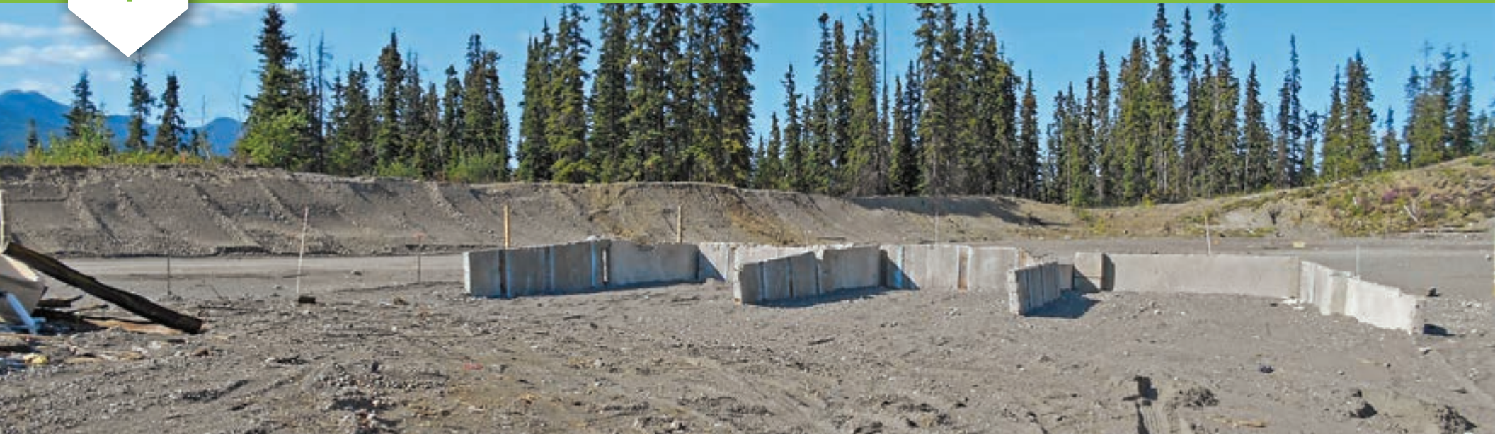
Improvements in progress at the Marsh Lake Solid Waste Facility.
