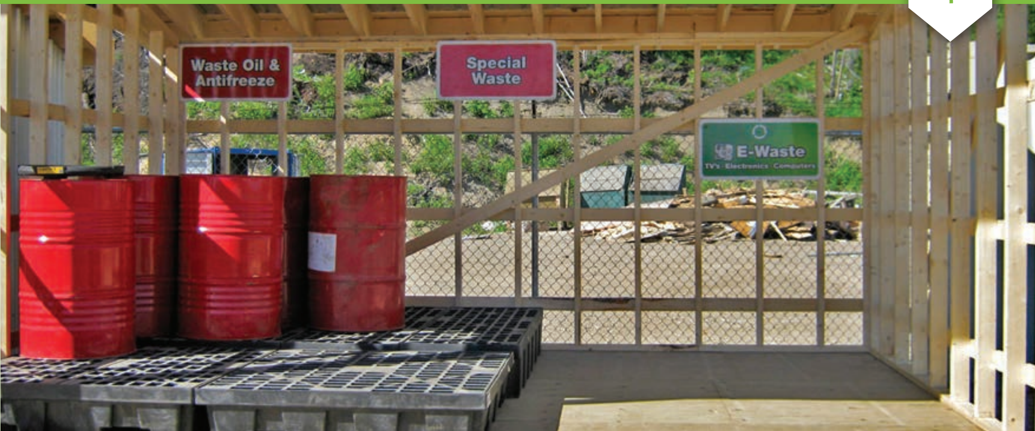
Household hazardous waste shed, Old Crow Solid Waste Facility.
