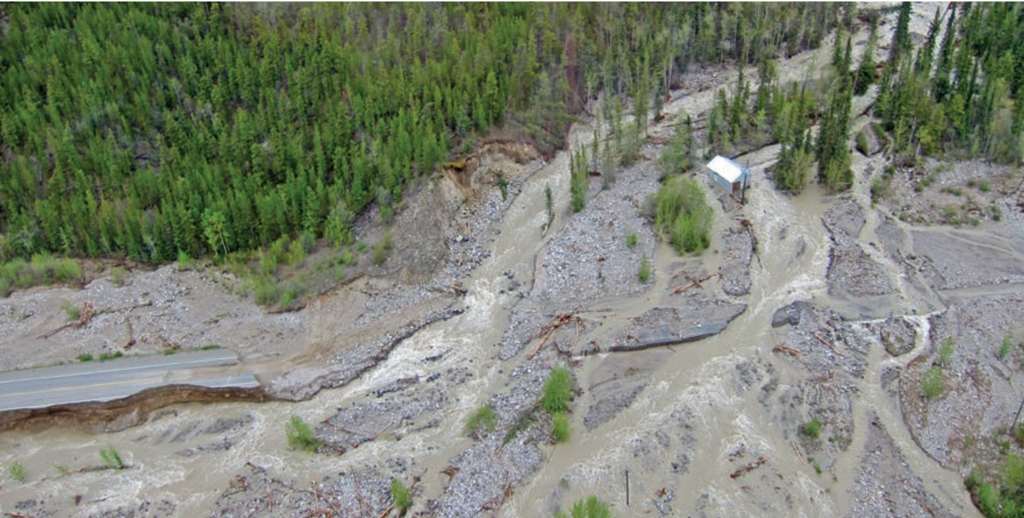
Flooding on the South Alaska Highway, Rancheria area, 2012.
