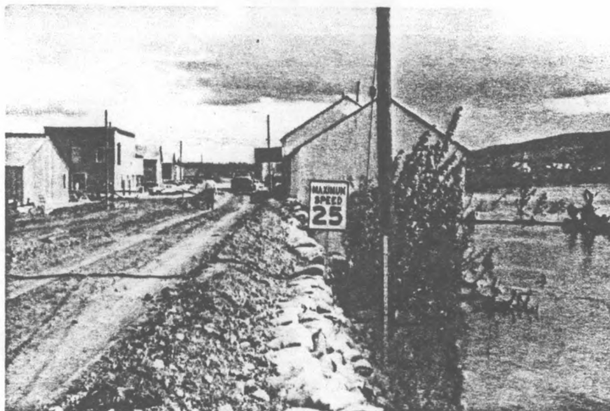
Fig. 9 - 1964 Flood Dike Construction.
