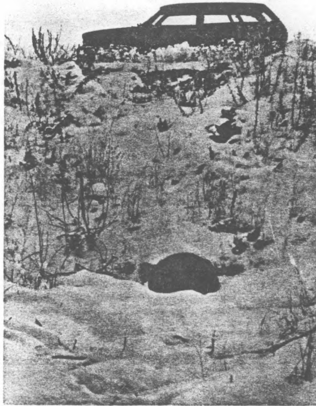
Fig. 15 - Drainage culvert through dike.
