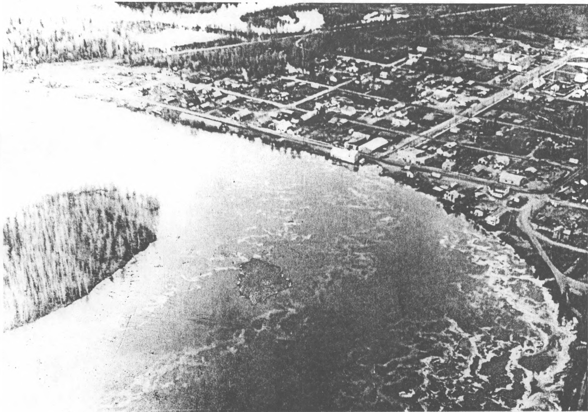
Fig. 7 - 1964 Flood - Aerial view of Mayo
