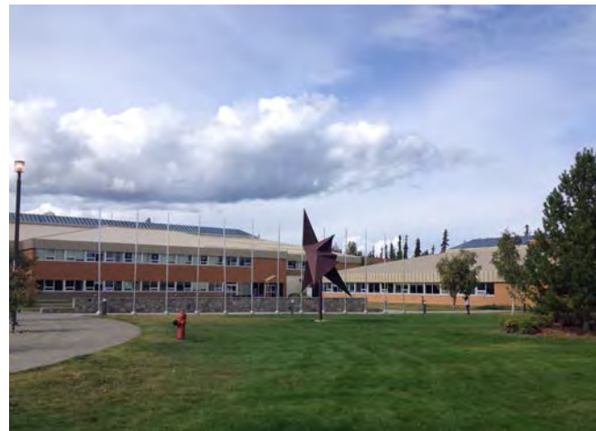
Figure 19 - View of central courtyard from the Yukon Archives building
