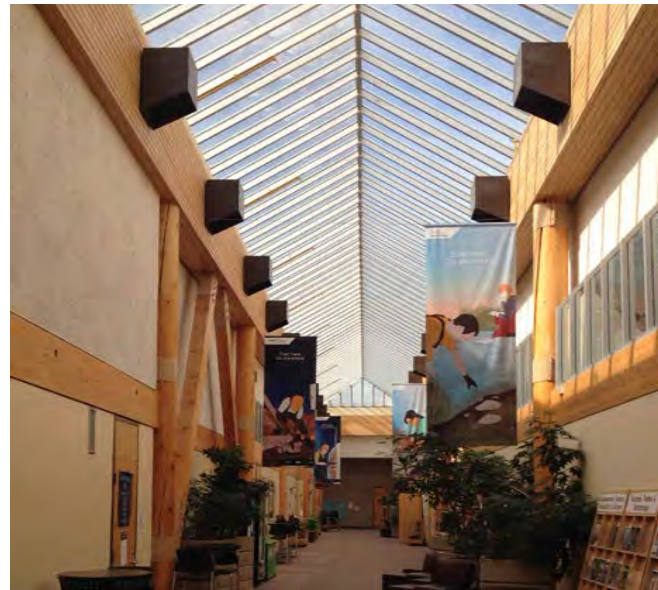
Figure 18 - Skylights provide daylight within the internal circulation networks of the a-, c-, and t-wings
