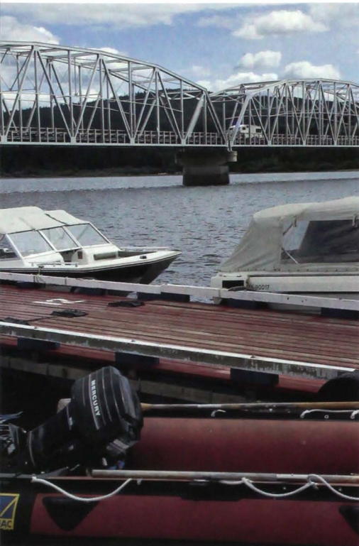
The Yukon's longest bridge spans the Teslin River at Teslin.
