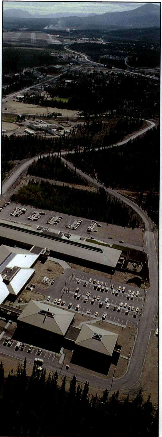
A bird's-eye view of the new Yukon College campus in Whitehorse and the site of the proposed Yukon Arts Centre.
