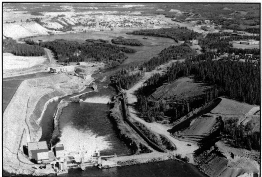
The Whitehorse Rapids Hydro plant was transferred from the federal government to the people of the Yukon through the Yukon Energy Corporation.
