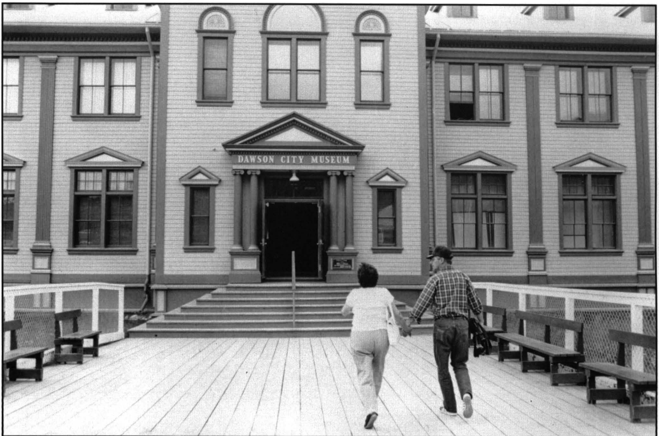
The department's Heritage Branch played a major role in the restoration of the Old Territorial Administration Building.
