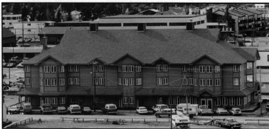
The Yukon Housing Corporation was responsible for ensuring that Closeleigh Manor is one of the best, and energy efficient, senior citizen housing units in the country.
