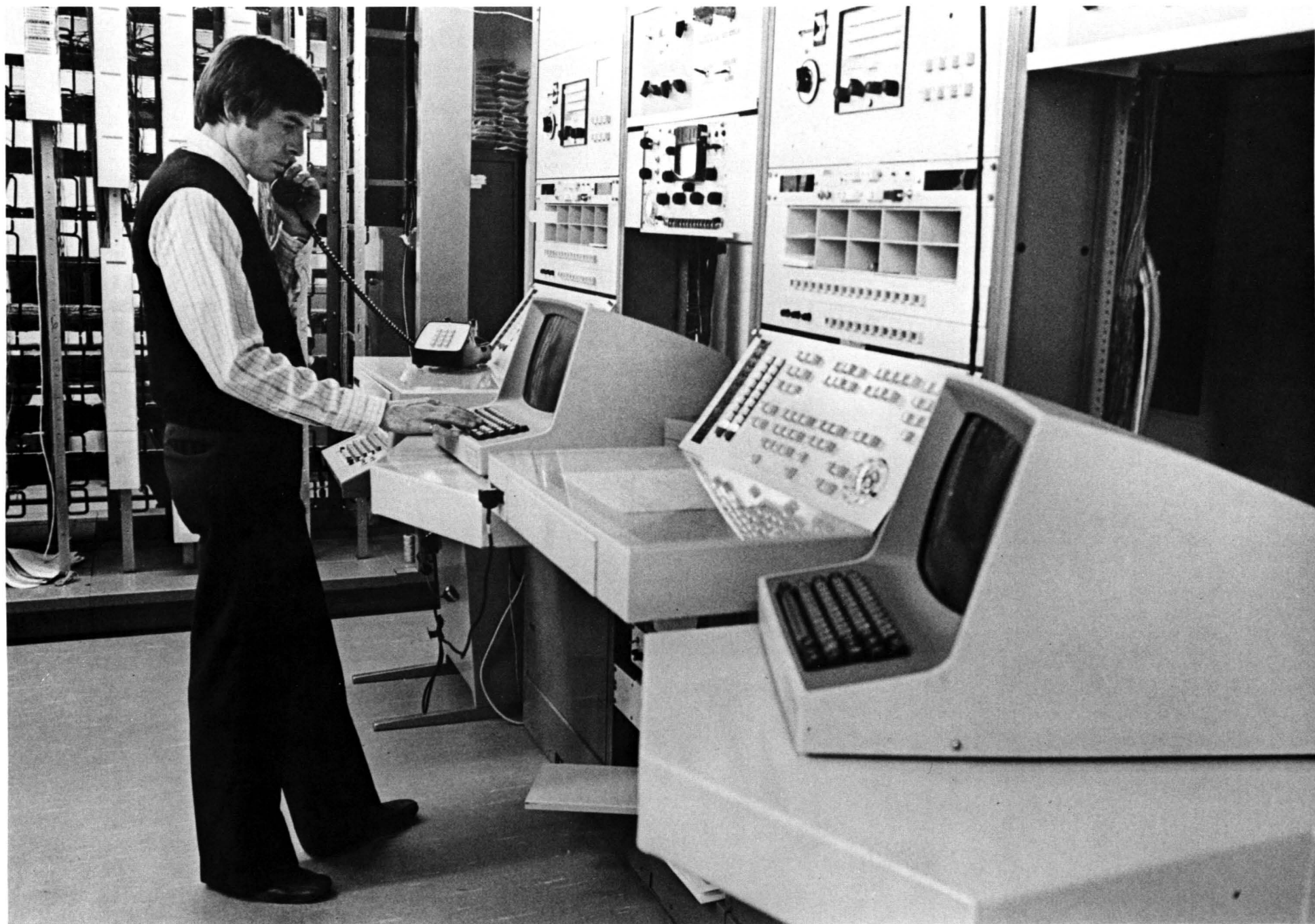
Installation of new Canadian National Telecommunications equipment in Whitehorse.
