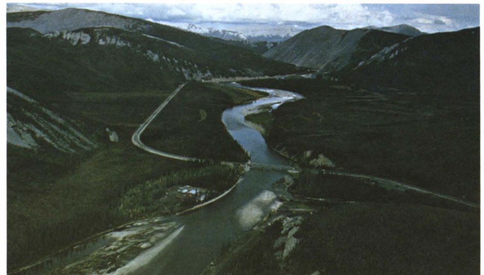
Ogilvie Bridge and maintenance camp on the Dempster Highway
