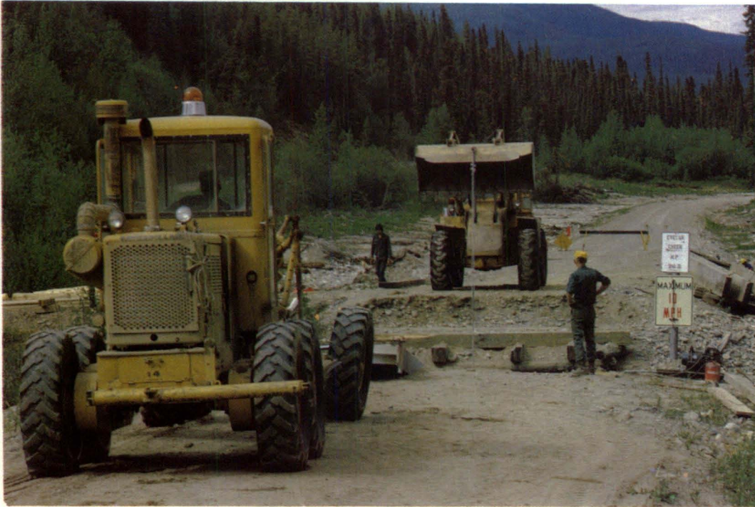
Highway Maintenance is a never ending task.
