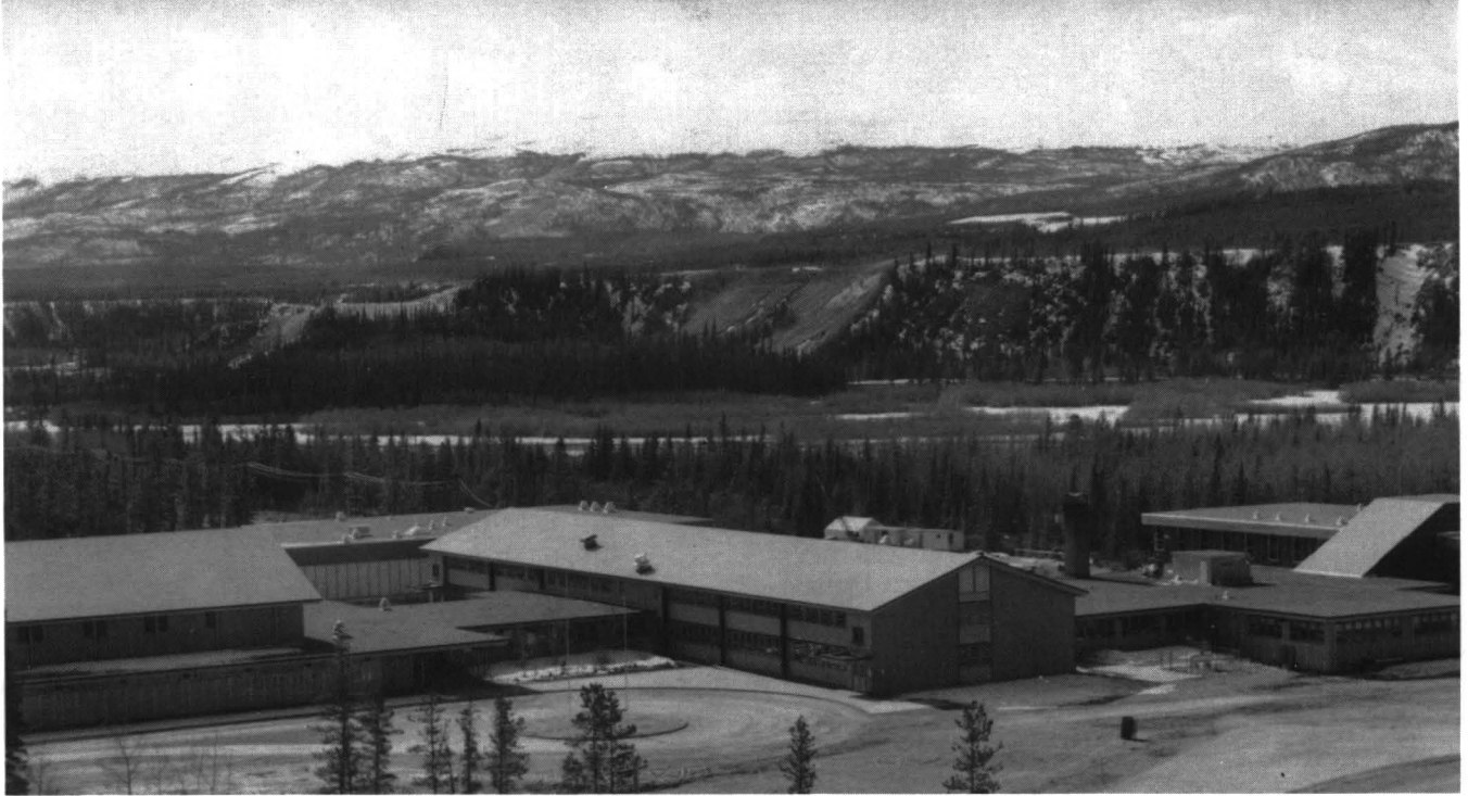
F. H. Collins Secondary School in Whitehorse.
