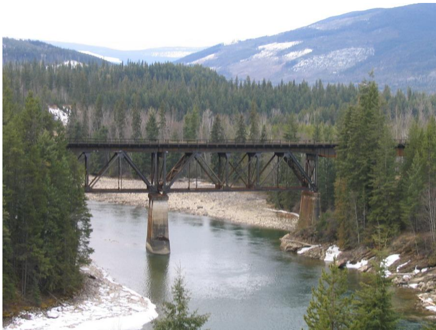
Picture 18: Large Bridge over River
