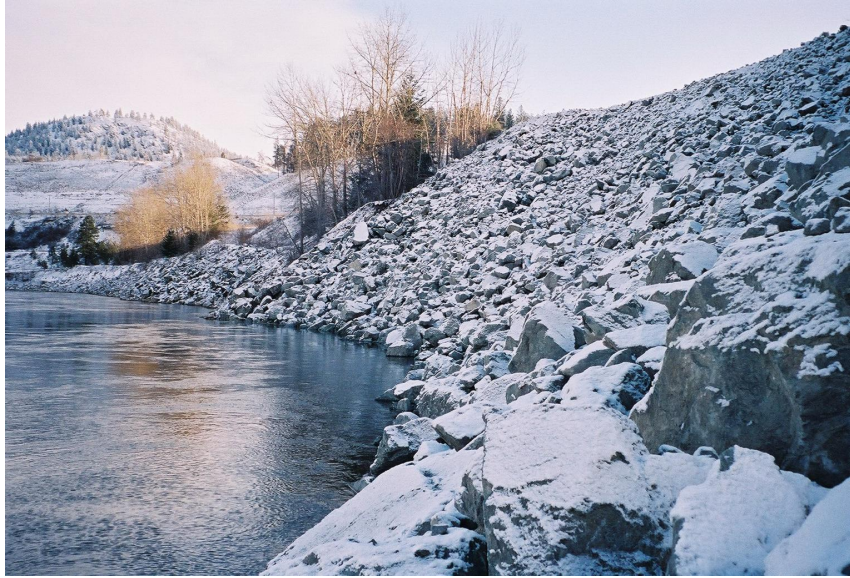
Picture 22: Riprap Erosion Protection
