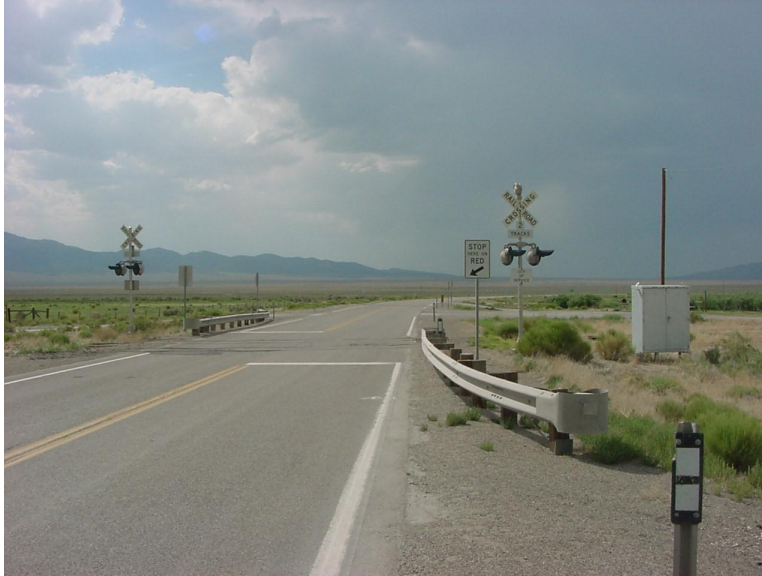
Picture 20: Level Road Crossing
