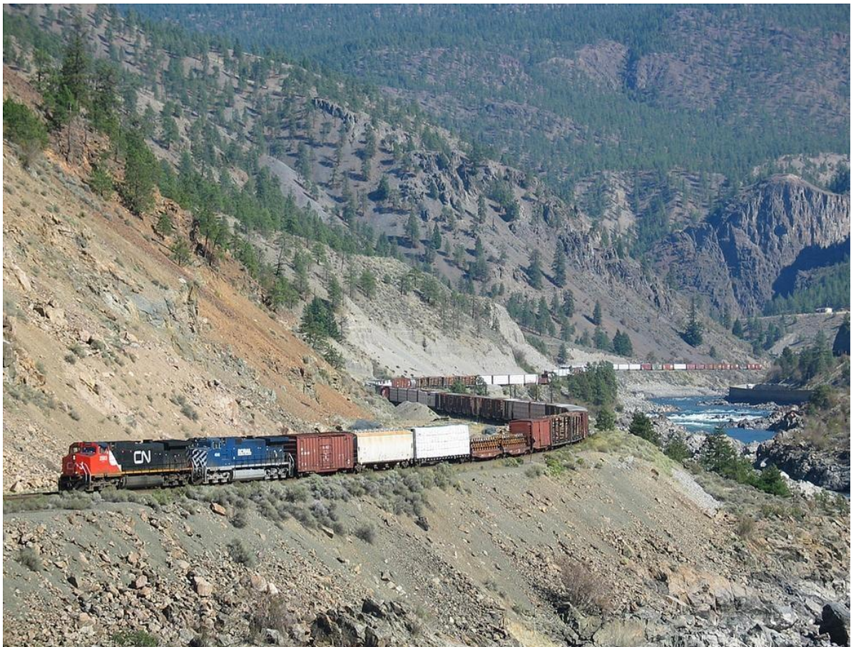
Picture 14: Very Heavy Grade Construction
