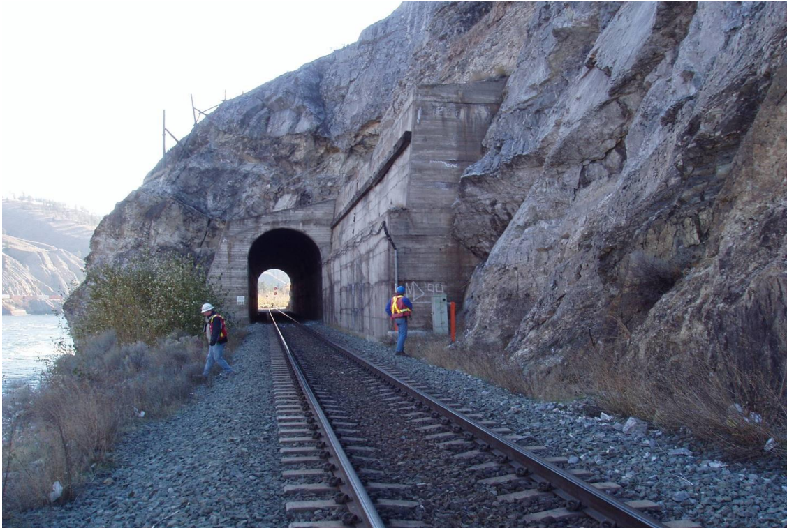
Picture 16: Short Tunnel and Buttress at Portal
