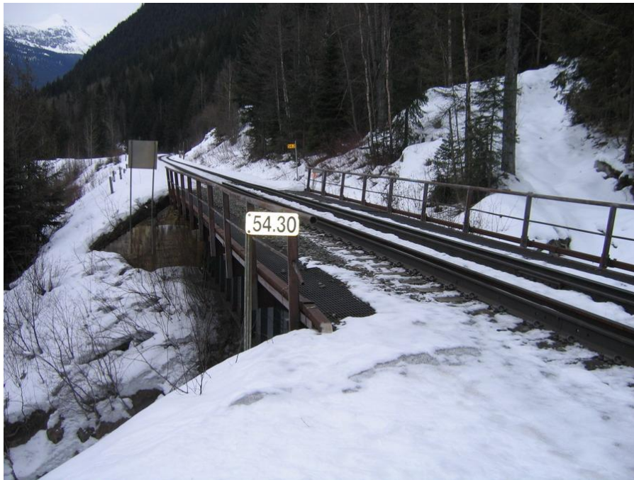
Picture 17: Small Bridge over Tributary
