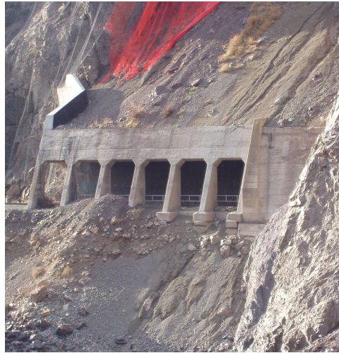
Picture 24: Rock Shed
