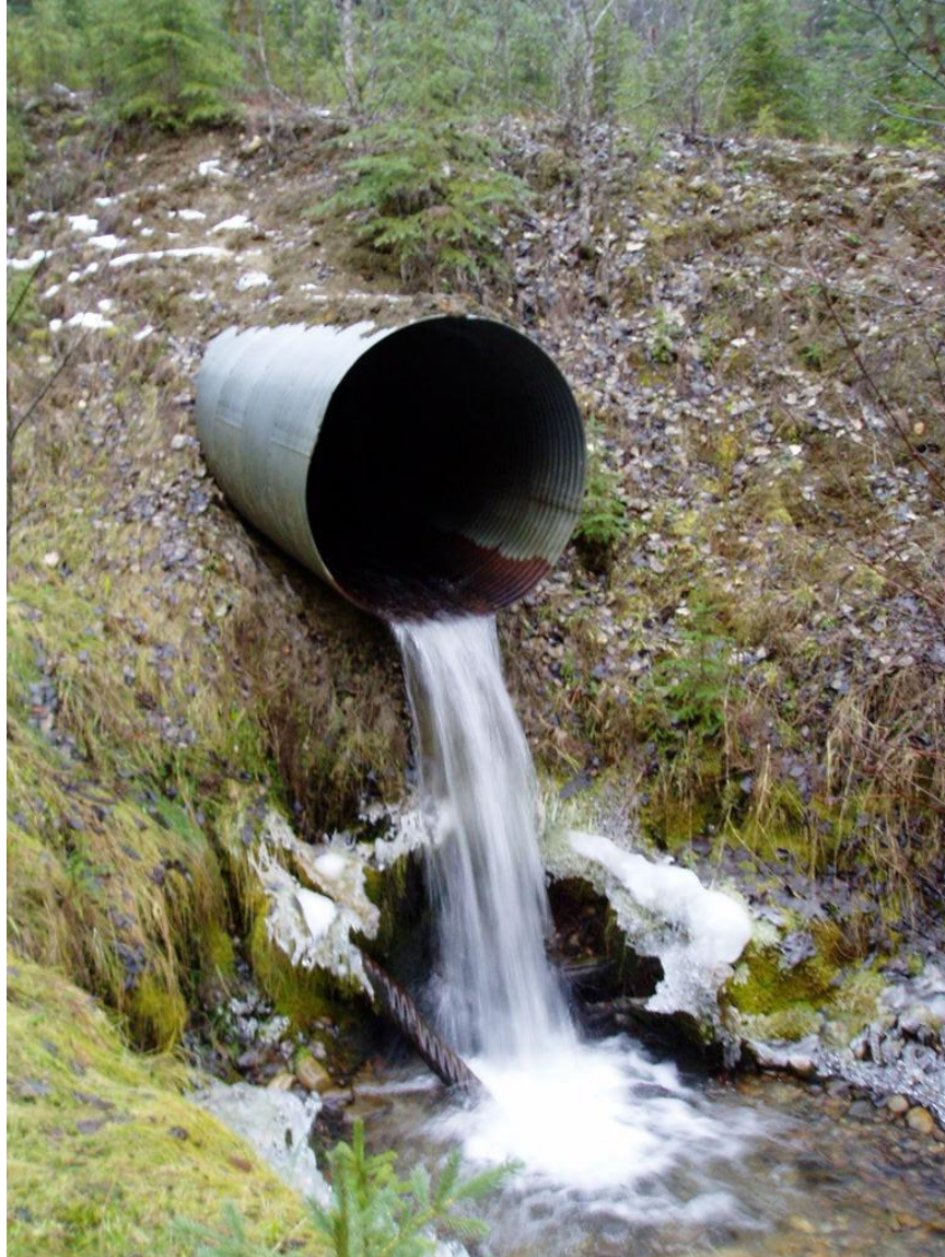
Picture 19: Bridge Pipe
