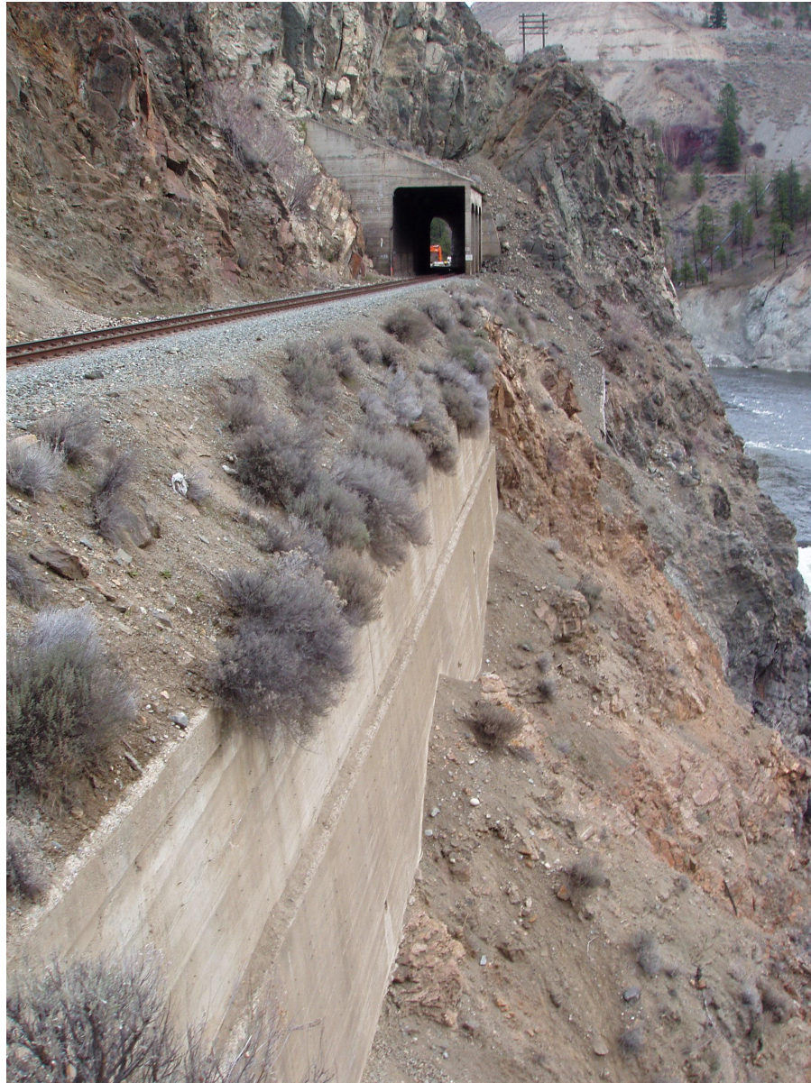
Picture 28: Concrete Retaining Wall
