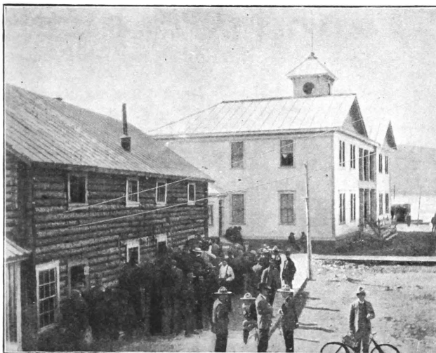
THE OLD LOG COURT-HOUSE AT DAWSON WAS JAMMED TO SUFFOCATION DURING THE HEARING OF THE CASE. [Photo.]
