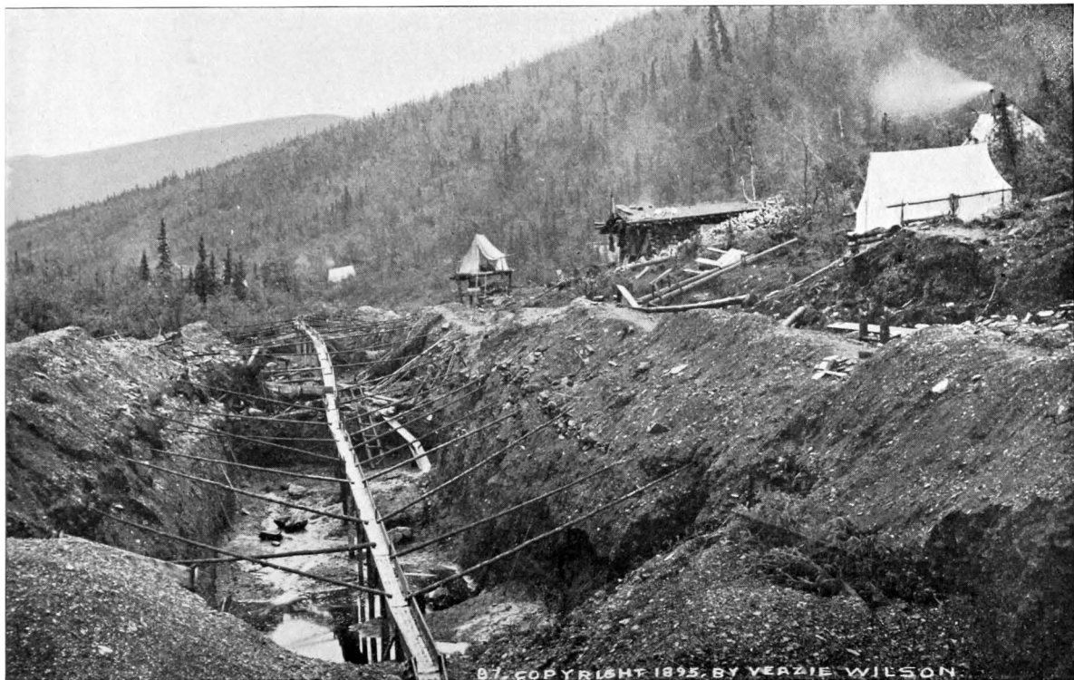
YOUNG AND BLANCHARD'S CLAIM AT MILLER CREEK. This shows the sluice boxes. This is a placer mine. Placer is a Spanish word and means, literally, pleasure, that is, plenty of metal easily mined.
