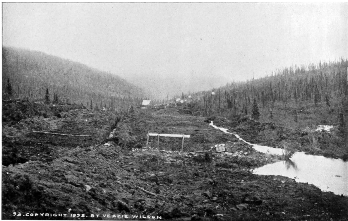
OPENING UP A CLAIM. The method of prospecting is usually carried on by sinking a number of holes to bed-rock across the bed of a creek, or cross cutting it by a tunnel and testing the dirt every few minutes.
