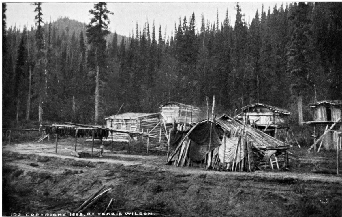
DRYING SALMON. Lower River. Showing caches. A cache is made by erecting a strong house upon posts twelve or fifteen feet above ground.
