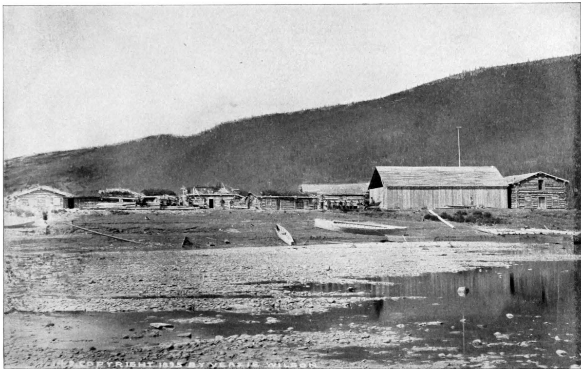
FORTY-MILE POST FROM THE YUKON. The buildings here are all of logs chinked with moss. The roofs are of poles covered with a layer of dirt.
