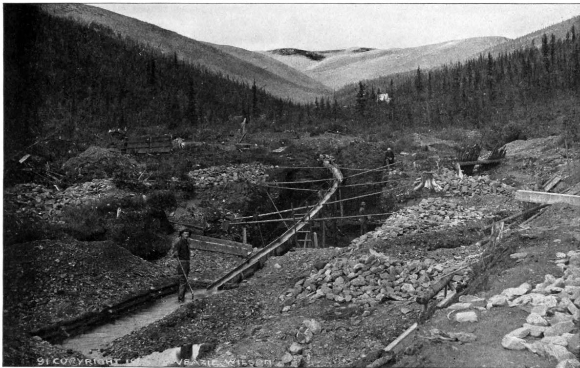
CLAIM FOUR ON MILLER CREEK. This shows the sluice, which is a long box with riffles. They are often joined in series and may extend several hundred feet.
