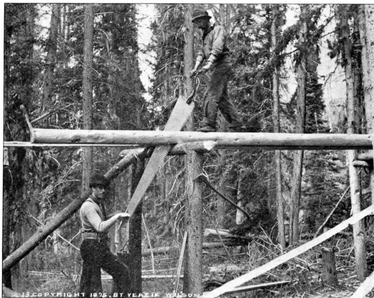
PRIMITIVE SAW MILL. Head of Lake Bennett. The timber has to be packed from where it is sawed to navigable water.
