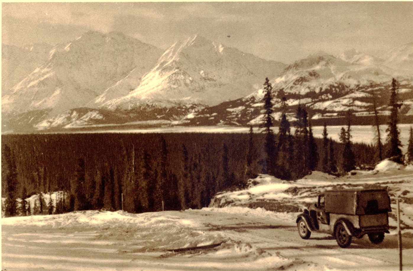
ON THE ALASKA HIGHWAY, OVERLOOKING THE SLIMS RIVER—TEMPORARY ROAD
