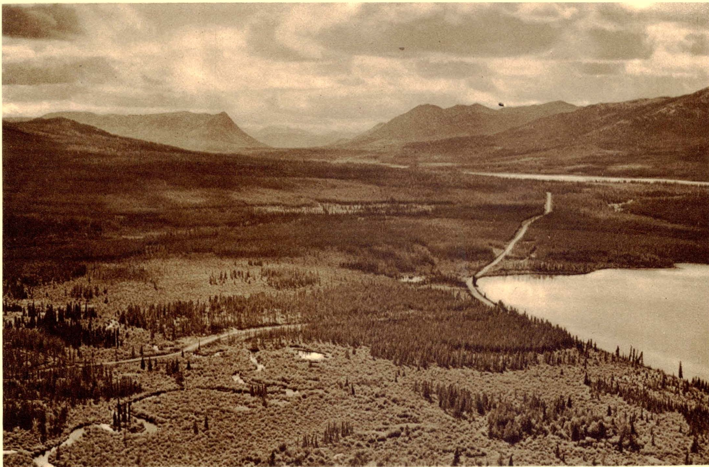
AERIAL VIEW OF PART OF THE ALASKA HIGHWAY
