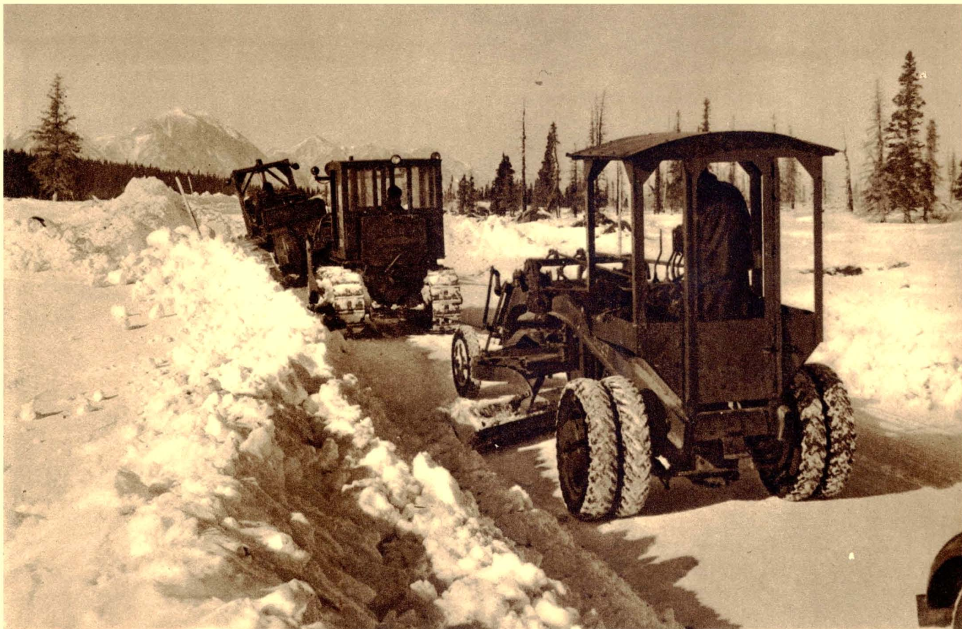
SNOW CLEARING ON THE ALASKA HIGHWAY NEAR BEAR CREEK SUMMIT, YUKON TERRITORY
