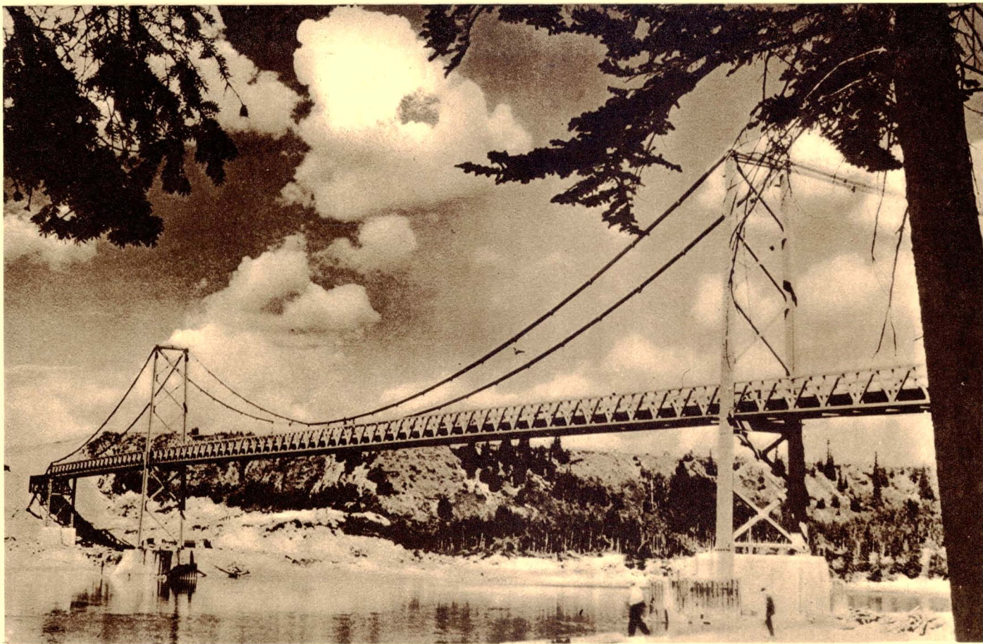
THE PEACE RIVER BRIDGE
