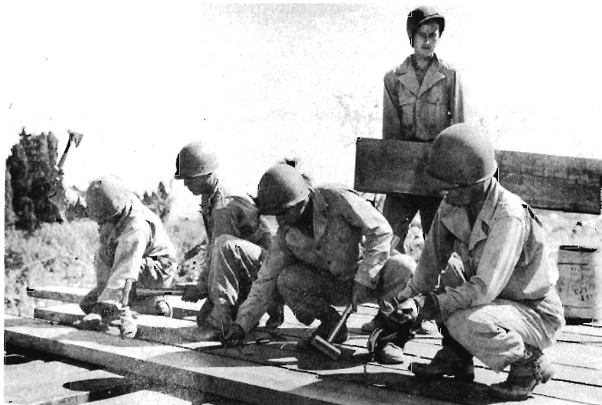
Figure 128. Nailing deck plank to timber stringers. The timber stringers shown are substitute-size shallow stringers.
