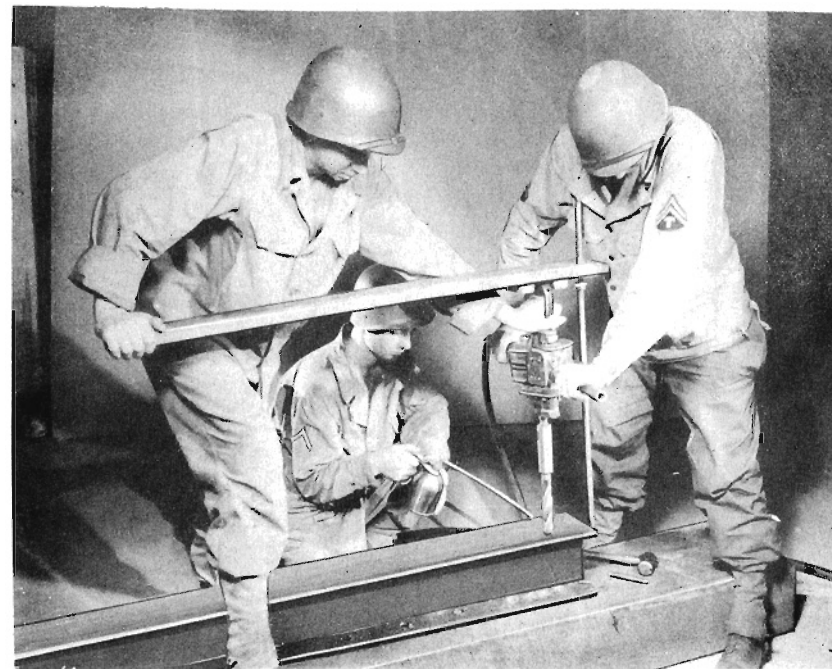
Figure 48. Drilling 15/16-inch holes in steel with the pneumatic wood borer.
