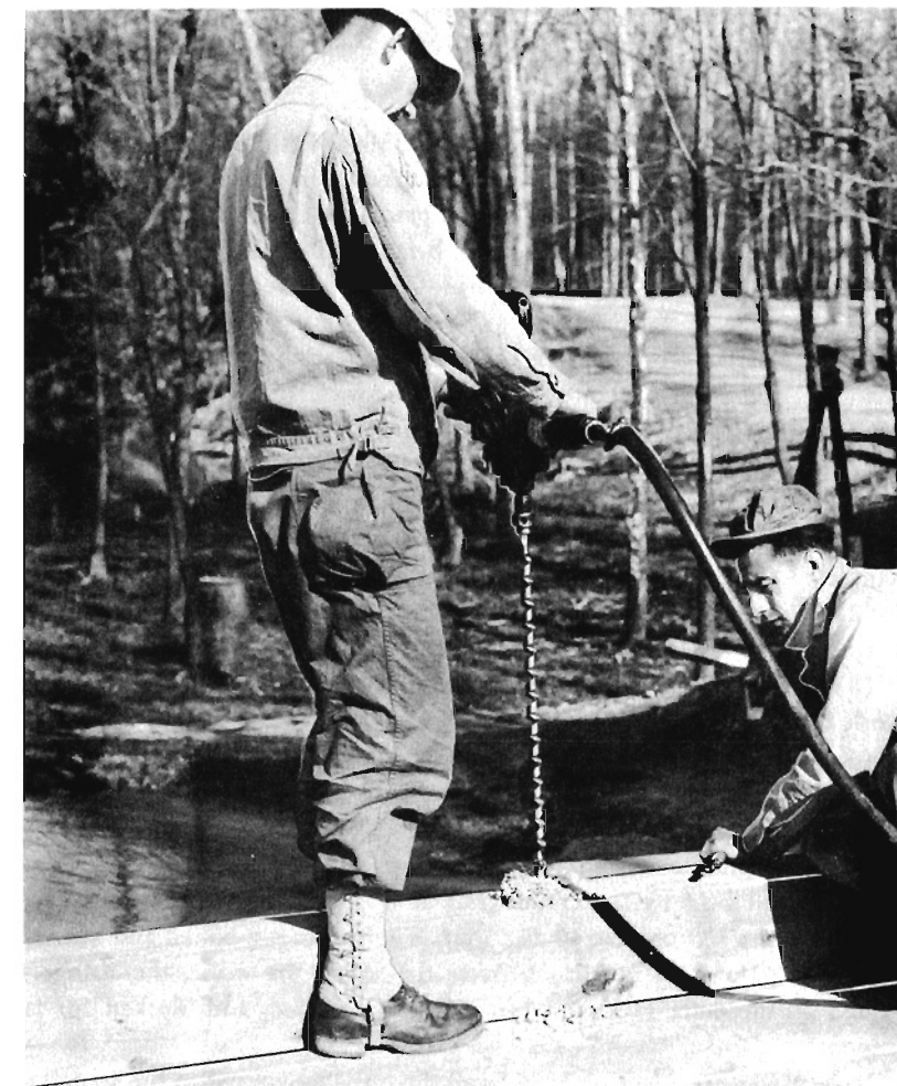
Figure 130. Drilling curb with pneumatic wood borer.
