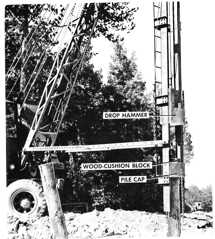
Figure 85. Standard drop hammer and pile cap.
