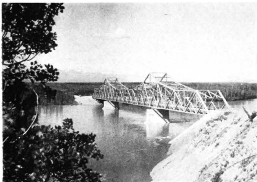
Figure 25.—The Highway bridges the Tanana.
