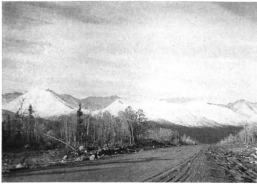
Figure 40.—Alaska Highway, ready for gravel surfacing.
