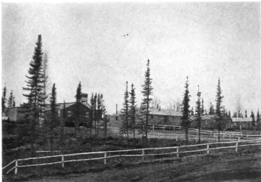
Figure 47.—One of the better construction camps, Alaska Highway.
