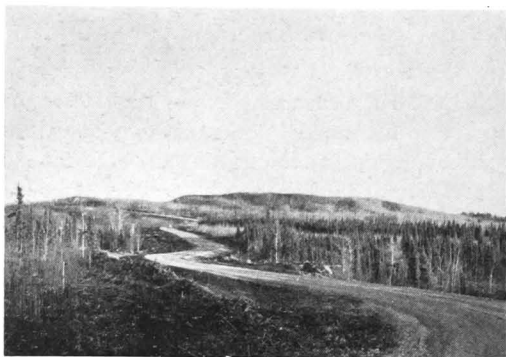
Figure 21.—Section of pioneer alignment retained, Alaska Highway.
