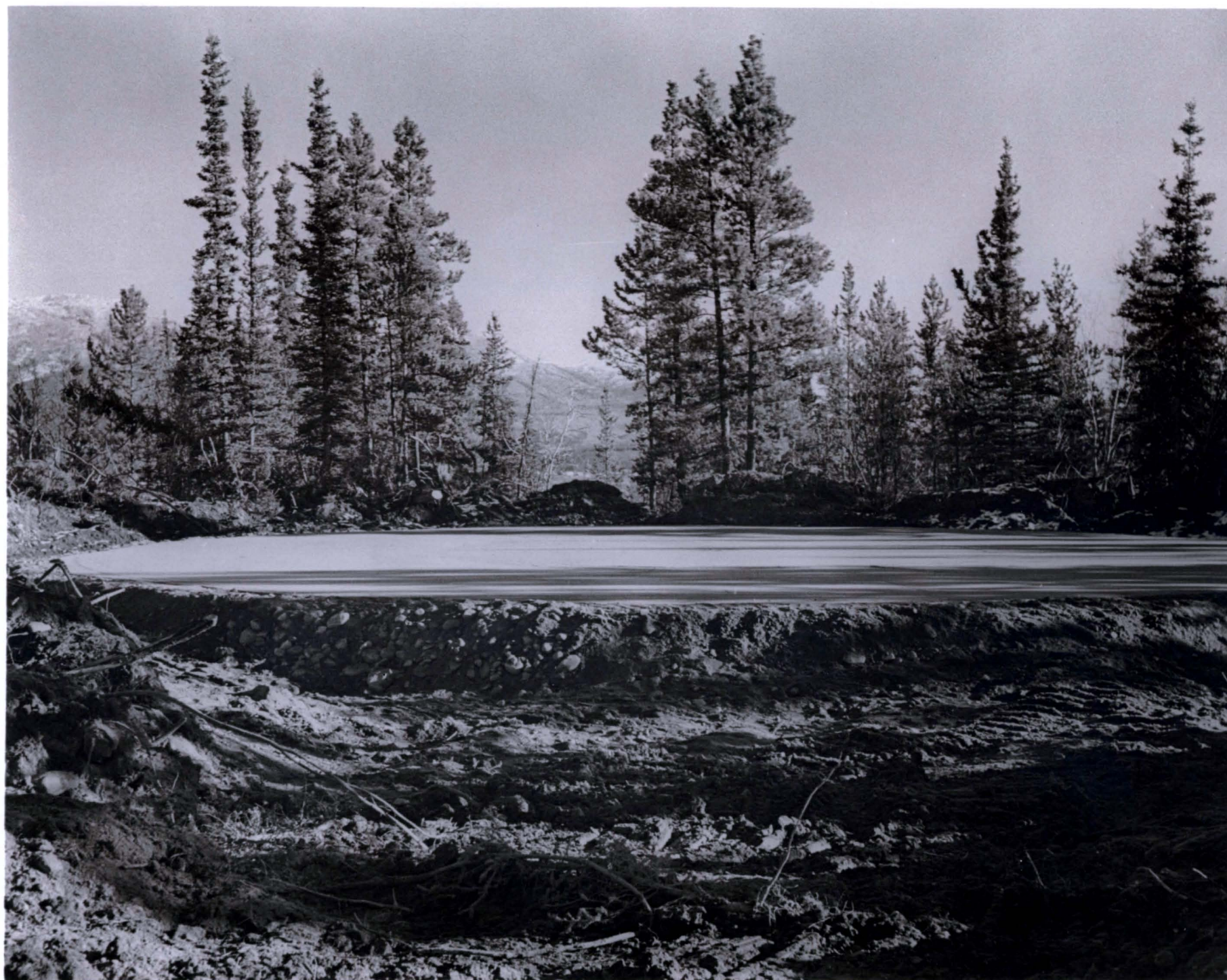
Tank Site No. 3 at Whitehorse ready for tank.
