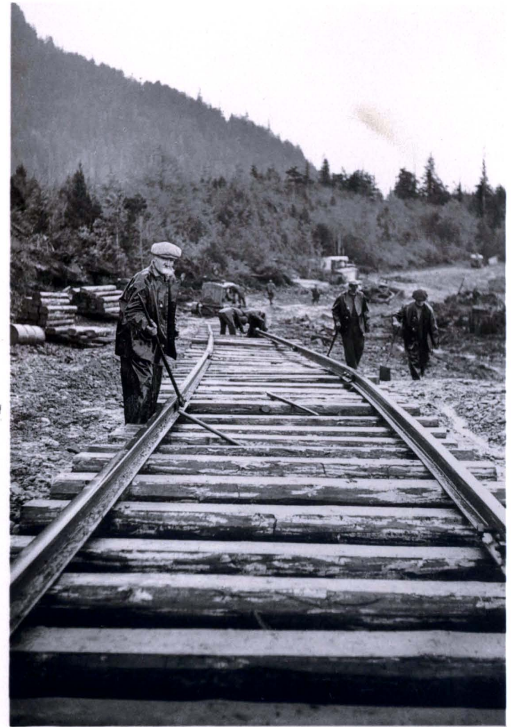
Railroad spur construction at Port Edward.
