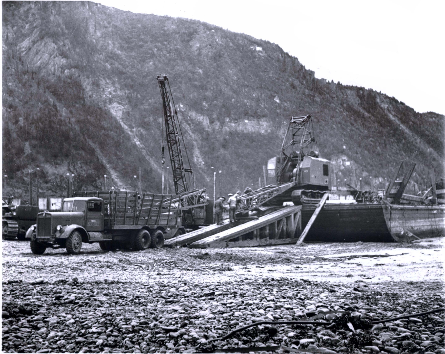
Crane being unloaded at Skagway. The barges are beached at low tide.
