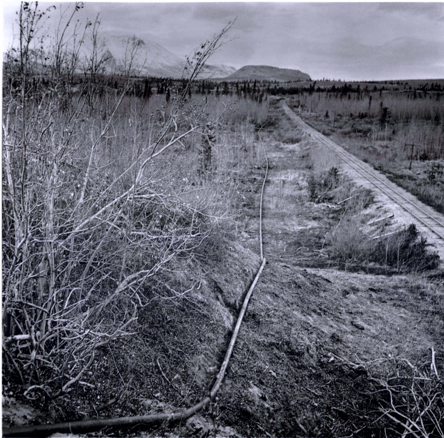
Welded pipe running northward along railroad 1 mile out of Carcross.
