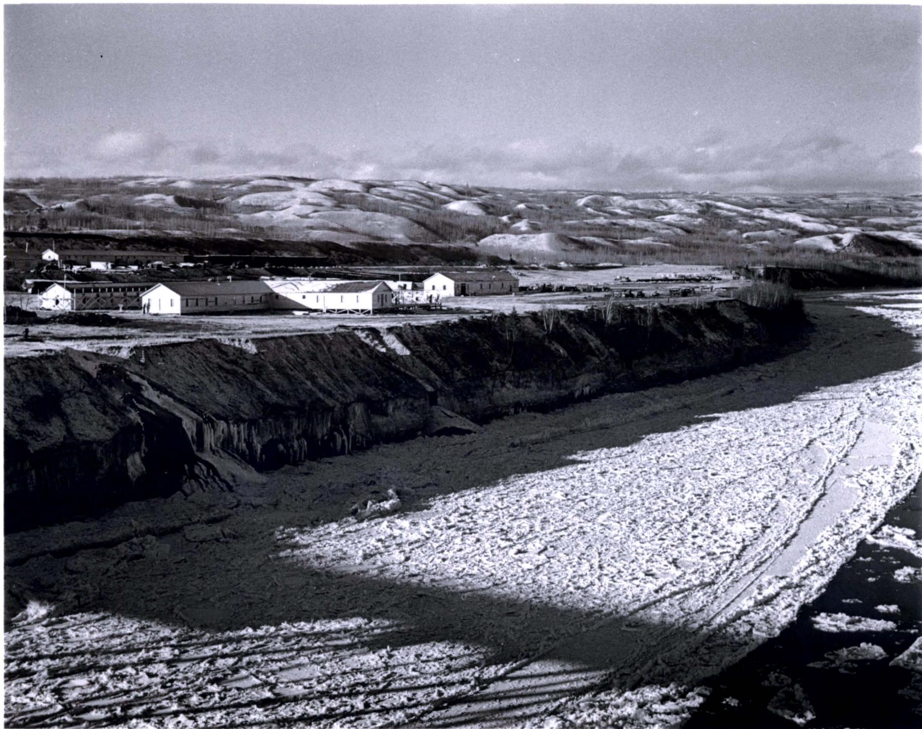
Constructor's base camp at Peace River.
