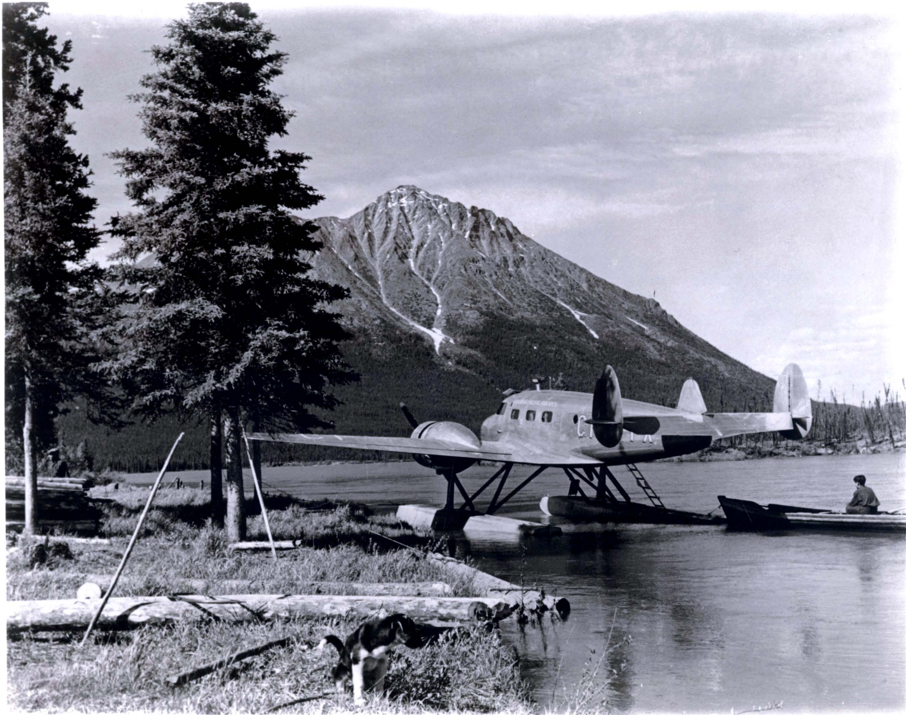
The first reconnaissance. BTX at Sheldon Lake.
