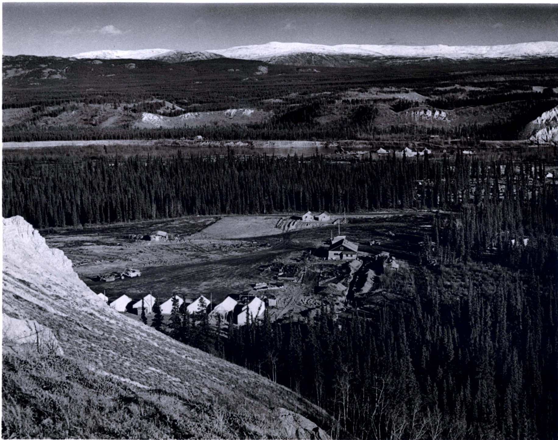
Constructor's camp seen from bench back of Whitehorse.
