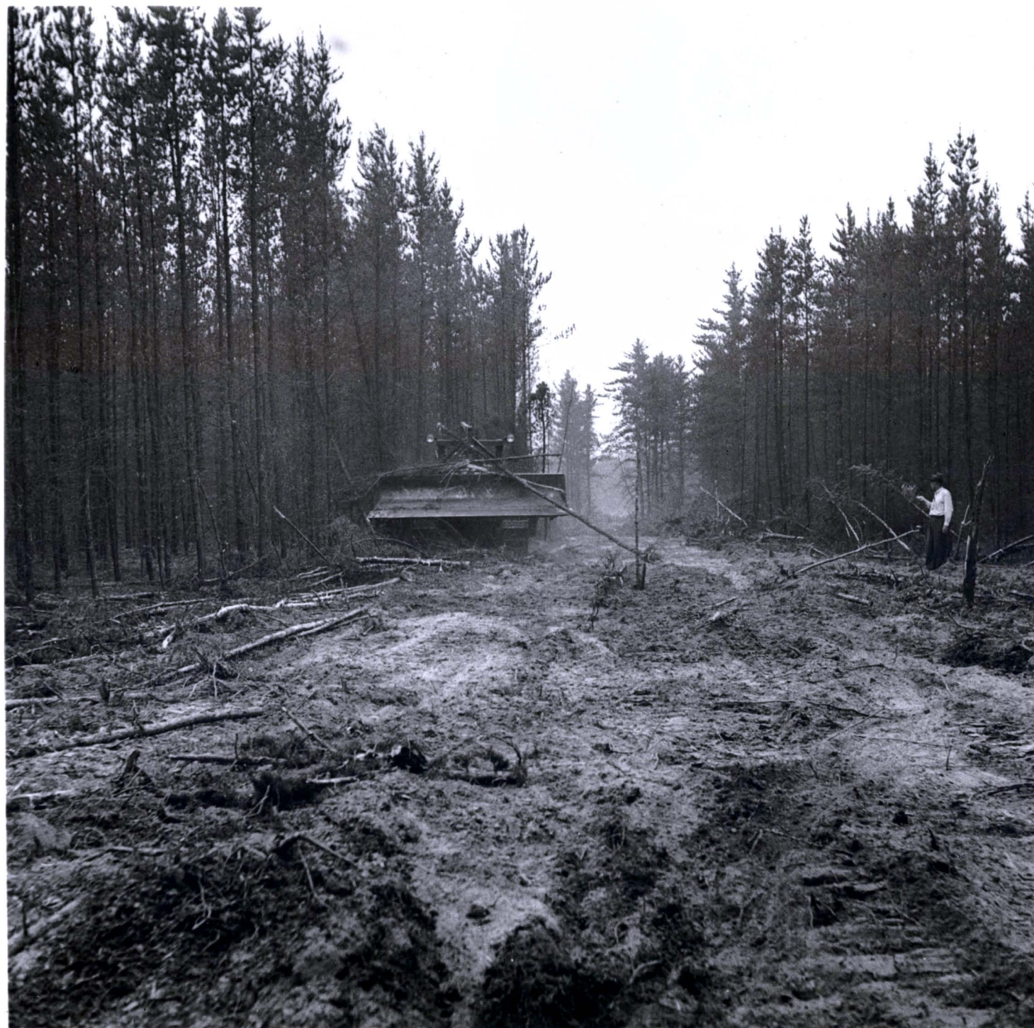
Bulldozer at work on one of nine airfields.
