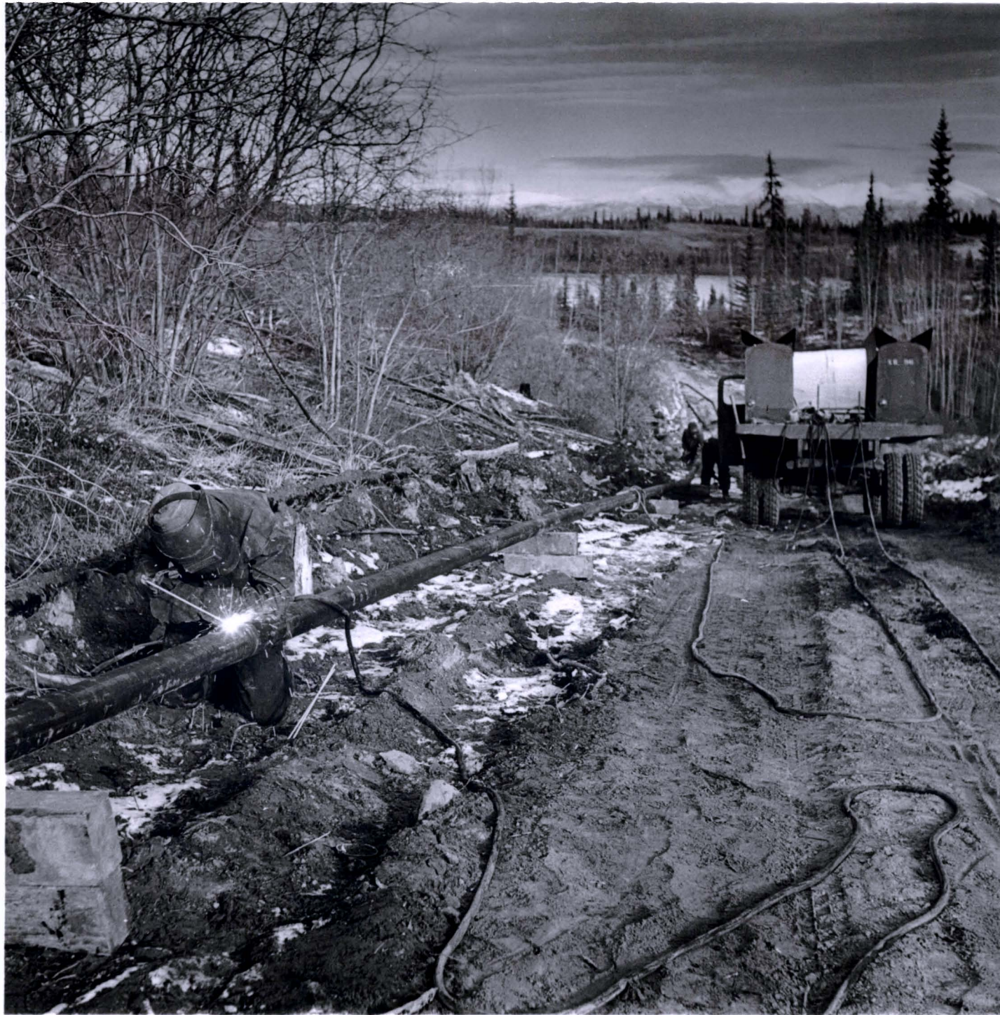
Welding between Mile 94 and Mile 95 north from Skagway.
