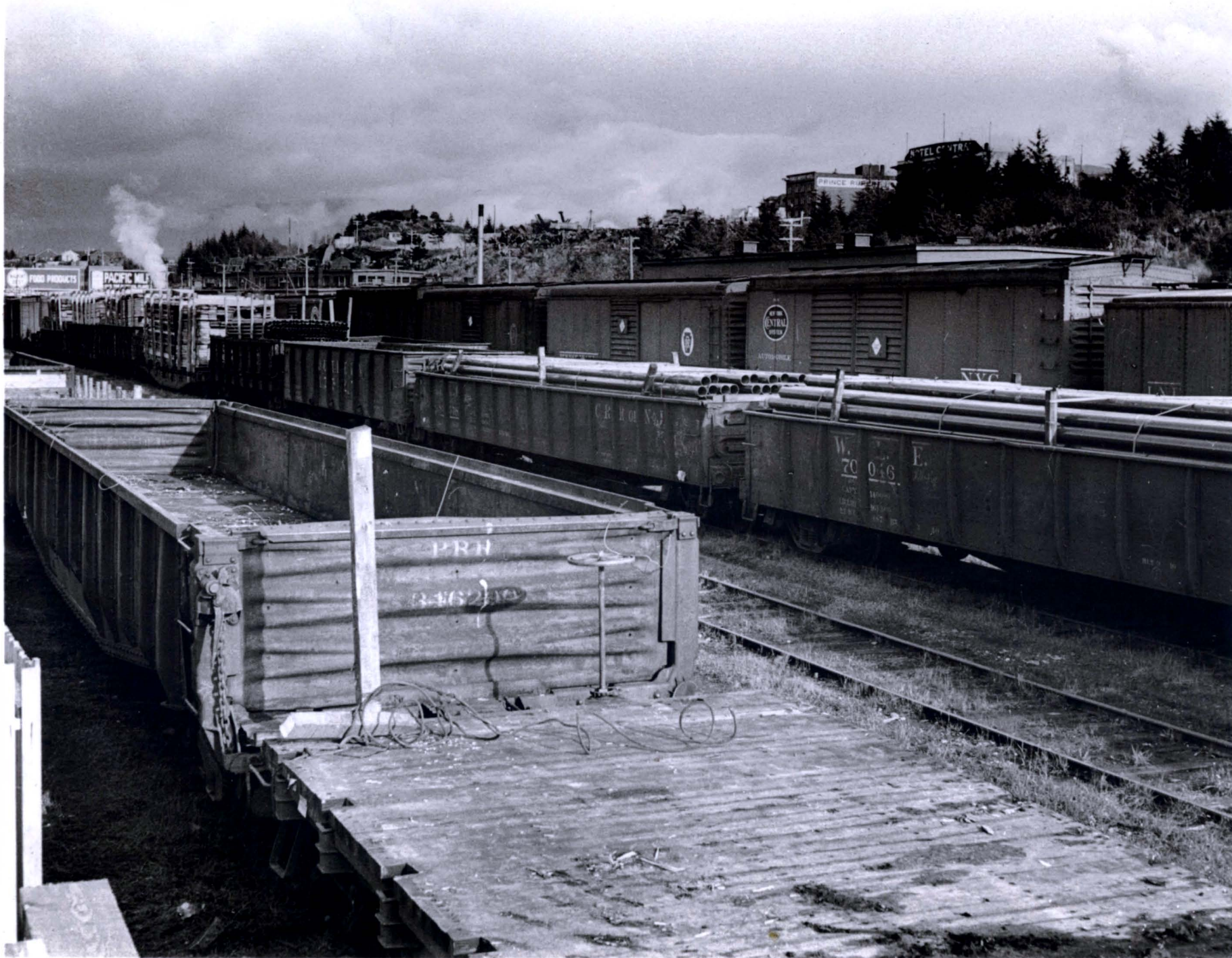
Carloads of six-inch pipe at Prince Rupert. It will travel by barge to Skagway and by narrow-gauge railroad to Carcross and Whitehorse.
