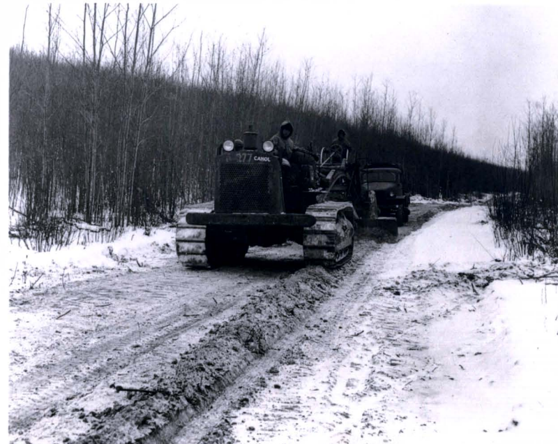
Tractor and grader on Grimshaw Road at Mile 115 from Peace River.
