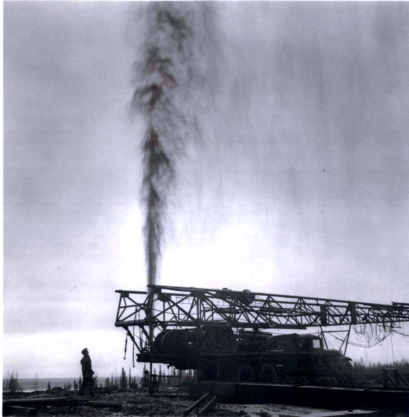
Blowing No. 18X at Norman Wells.
