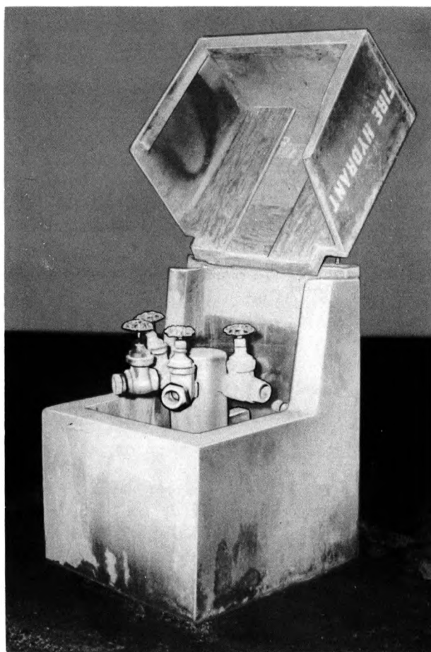
FIGURE 2F2-2 Hydrant Box Opened To Show Hose Connections
