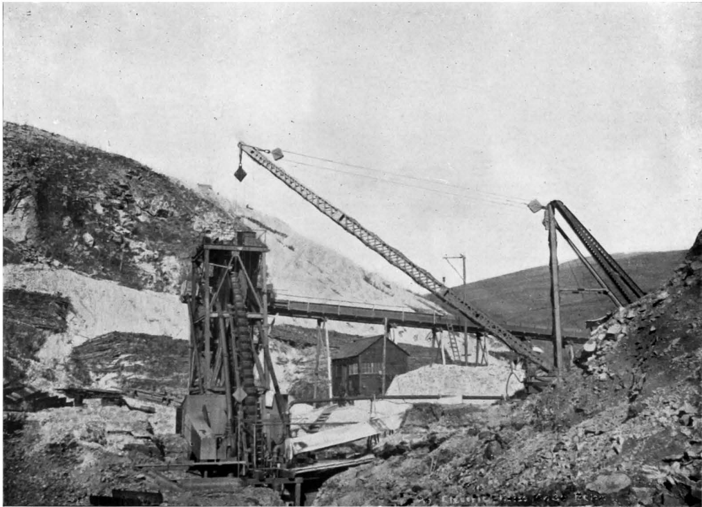
AN ELECTRIC HOIST ON 30 BELOW, BONANZA, Y. G. CO.
