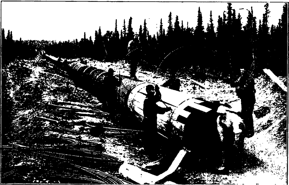
CONSTRUCTING STAVE-PIPE ON LEPINE RIDGE.
