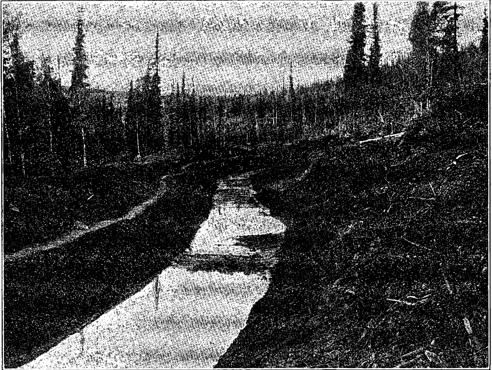
FINISHED DITCH, BEFORE WATER IS ADMITTED.
