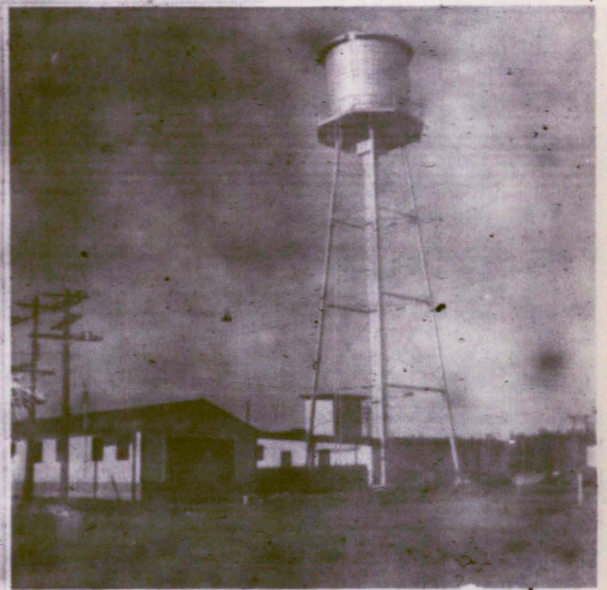
Muskwa Garr. Firehall Constructed 1957
