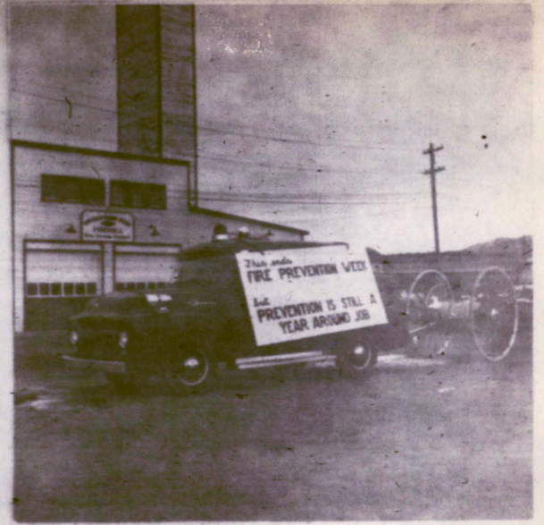
No. 1 Firehall - Bldg. F33 Declared Surplus 1962
