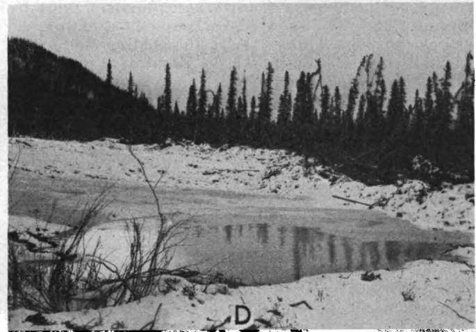
A, ICING STARTED AT ROADWAY EARLY IN THE WINTER. STRIPPING AN AREA ACROSS THE WATERCOURSE AT THIS POINT INDUCED ICING AND PROTECTED THE ROADWAY FOR THE REMAINDER OF THE WINTER. B, AN INDUCED-ICING AREA MADE WITH A BULLDOZER. C, A BUILDING PLACED OVER THE CULVERT INLET TO INCREASE HEATING EFFICIENCY. D, STORAGE OF ICE AND WATER AT AN INDUCED-ICING AREA.
