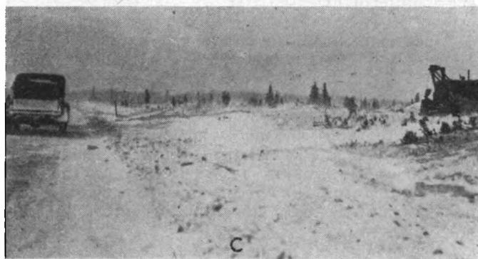
A, PERMAFROST EXPOSED BY GRADING IN ALASKA. B, WEST OF TANACROSS WHERE A "FROST DAM" FORMED AT THE ROADWAY. HYDROSTATIC PRESSURE HAS TIPPED THE TREES FROM VERTICAL POSITION. NOTE THE WATER ON THE SURFACE. C, AT THE SAME LOCATION AS B. HYDROSTATIC PRESSURE HAS RAISED THE THICK VEGETAL COVER AT THE RIGHT ABOUT 6 FEET.
