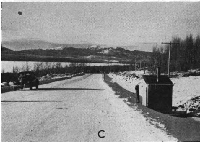
A, ICING STARTED AT ROADWAY EARLY IN THE WINTER. STRIPPING AN AREA ACROSS THE WATERCOURSE AT THIS POINT INDUCED ICING AND PROTECTED THE ROADWAY FOR THE REMAINDER OF THE WINTER. B, AN INDUCED-ICING AREA MADE WITH A BULLDOZER. C, A BUILDING PLACED OVER THE CULVERT INLET TO INCREASE HEATING EFFICIENCY. D, STORAGE OF ICE AND WATER AT AN INDUCED-ICING AREA.
