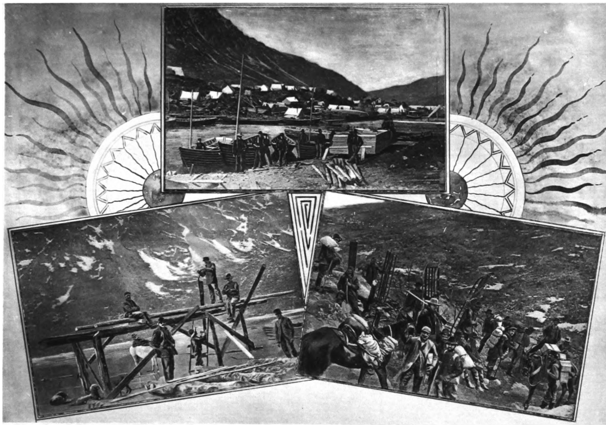
BOAT BUILDING AT LAKE BENNETT.
