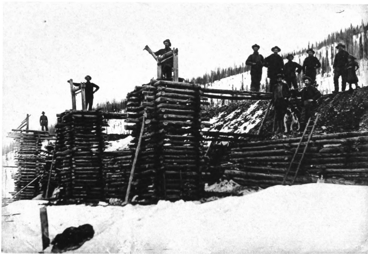
HIGH CRIBBING AT NO. 30 AND NO. 31 ELDORADO.
