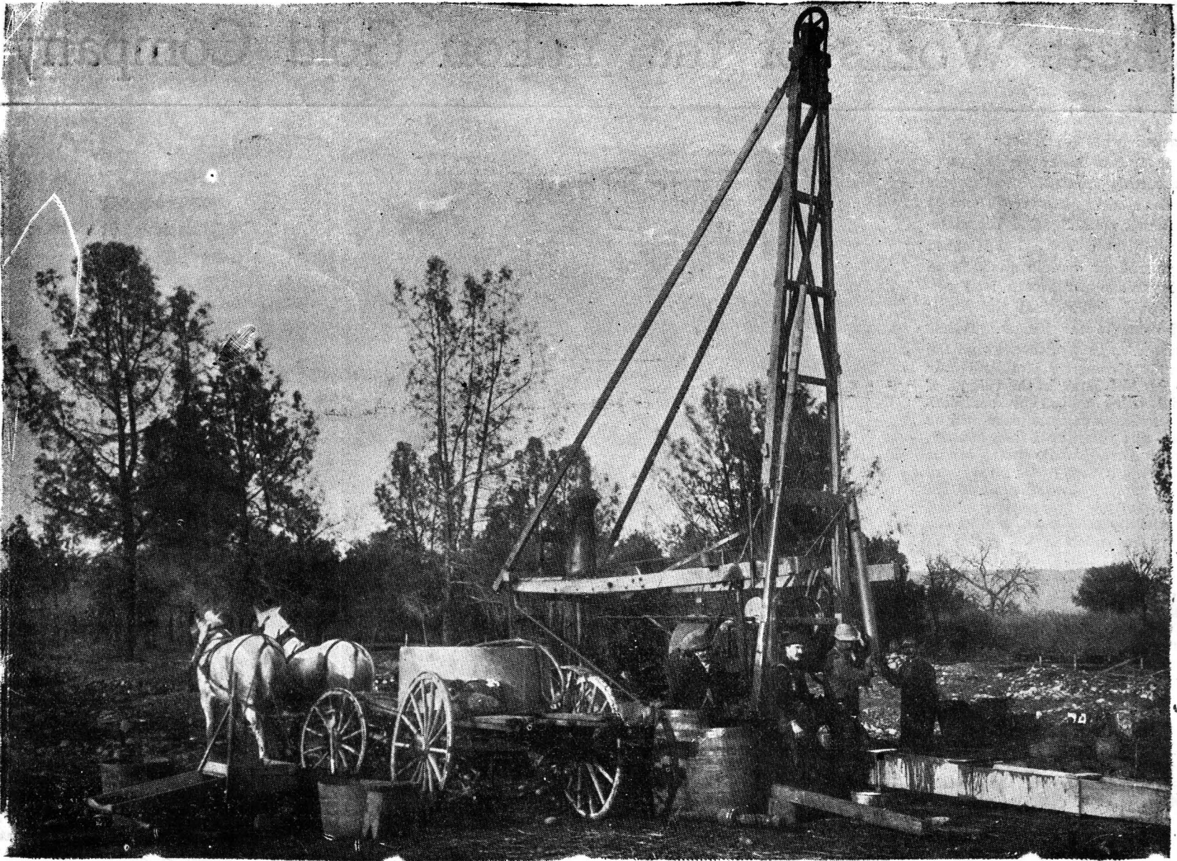
Testing Ground With Keystone Drill
