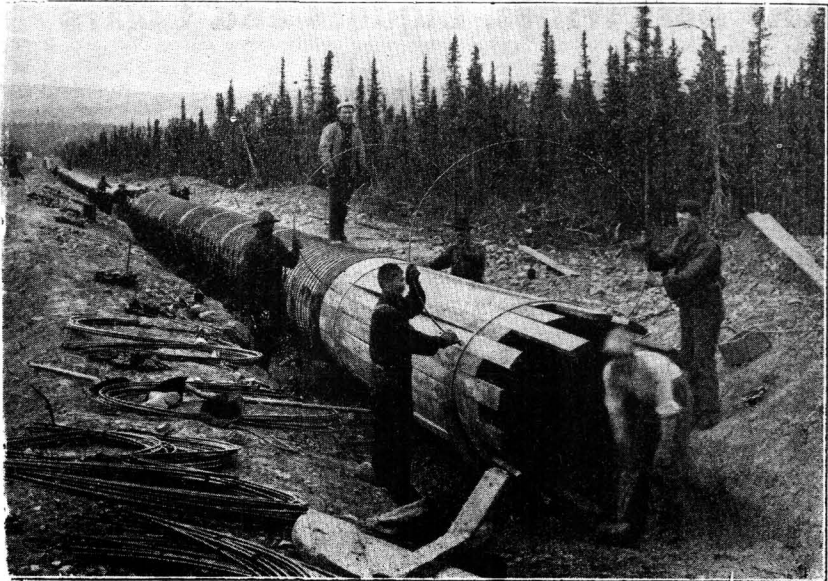
Building Pipe Line for Yukon Gold Hydraulics
