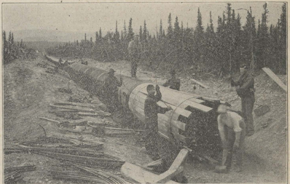
Wooden Pipe Line Under Construction.
