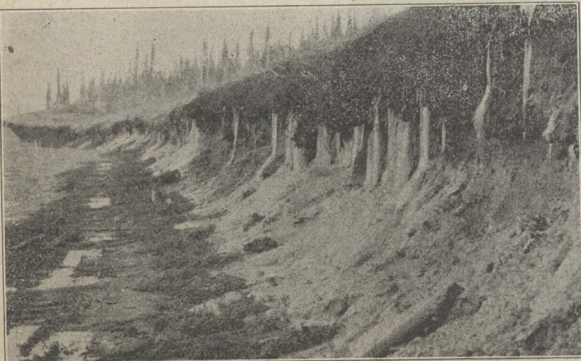
On the Line of Ditch.
