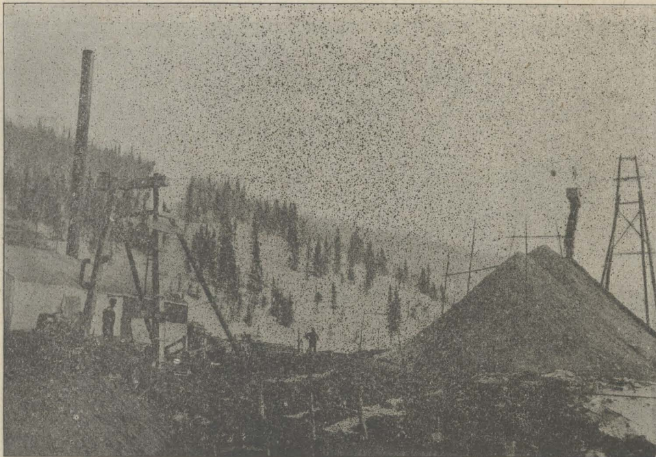
Drifting and Hoisting by Machinery.
