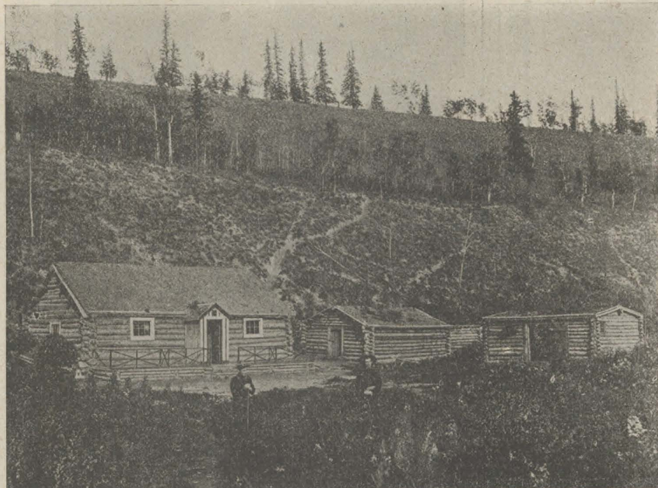
Hootchiku Police Station.
