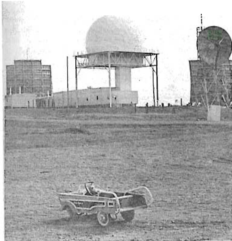
BAR-1 DEWLine Auxiliary Station in 1972.
