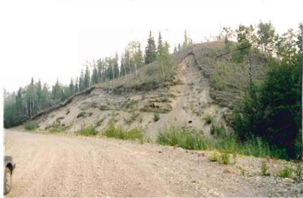
Figure 1.6. Esker at the Tatchun River culvert near Kelly Creek.
