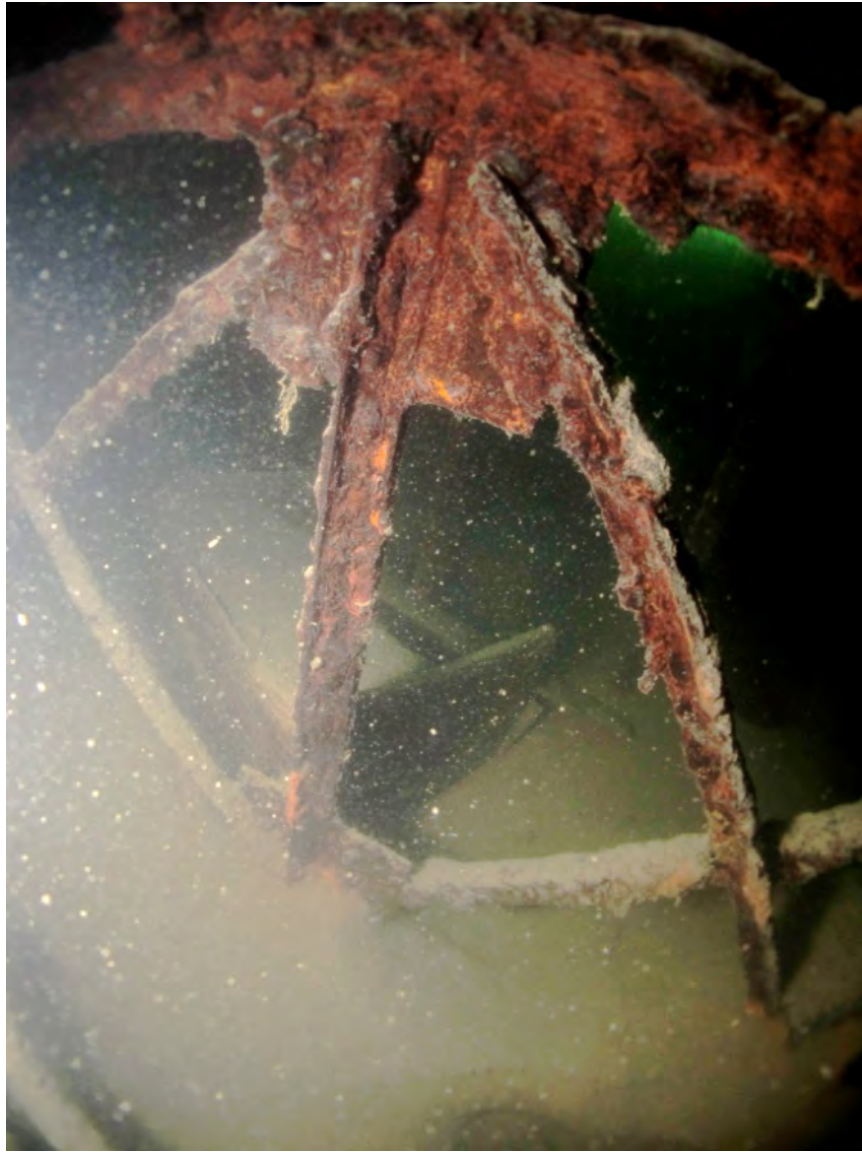
FIGURE 5.15. Diagonal trusses inside the hold (Photo by Geoff Bell).
