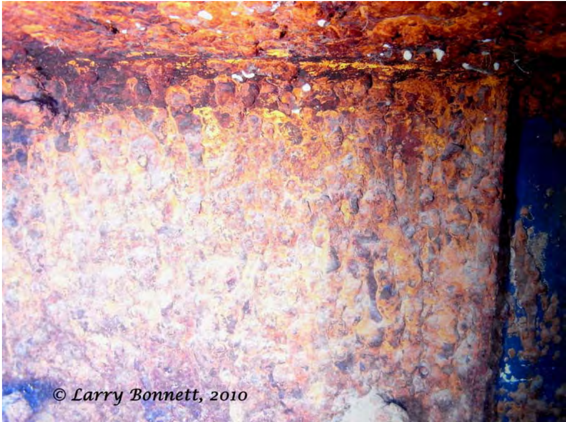
FIGURE 5.16. 2 in. (5.08 cm) angle iron clamp underneath deck (Photo by Larry Bonnett).
