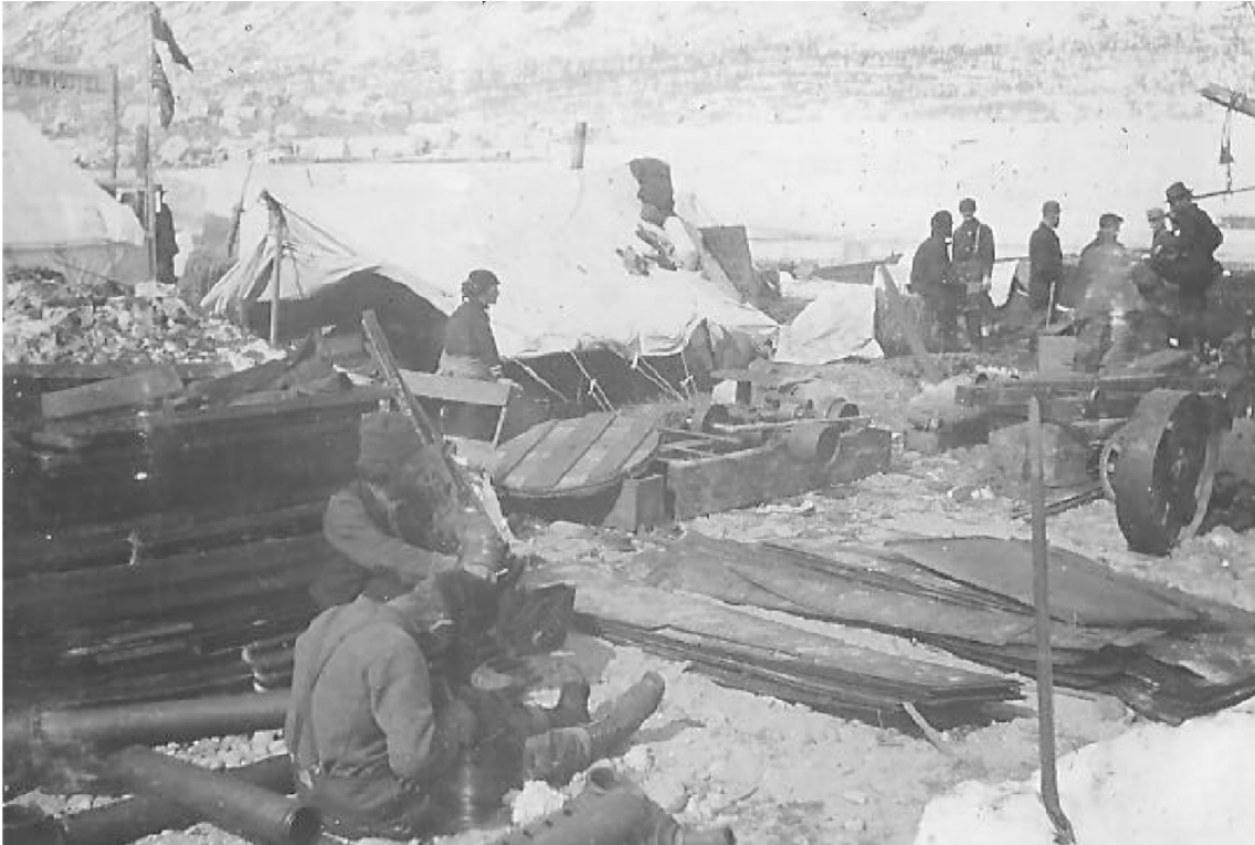
FIGURE 3.12. The steamboats A.J. Goddard and F.H. Kilbourne being assembled at Lake Bennett (Goddard collection, courtesy of Fay Goddard).
