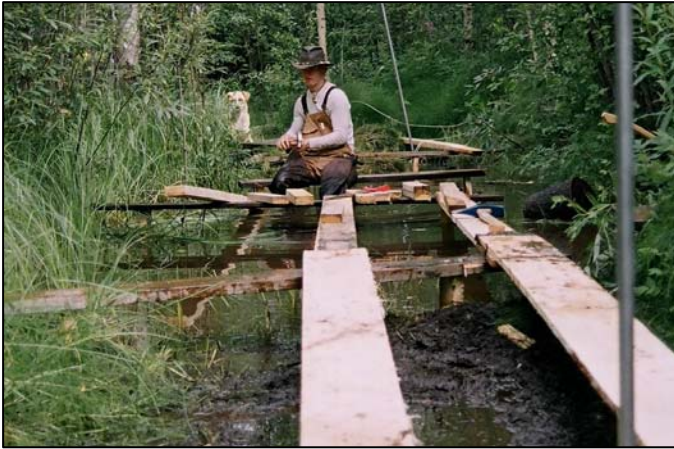
Constructing board walks along net lanes
