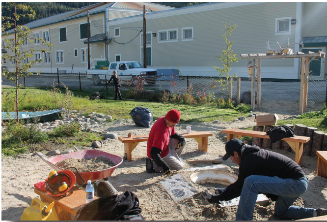
The WOP Crew puts the finishing touches on the Outdoor Classroom.
