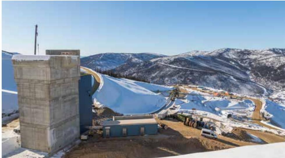
» Above: The primary crusher and coarse ore conveying storage on site at Victoria Gold's Eagle Gold mine.
