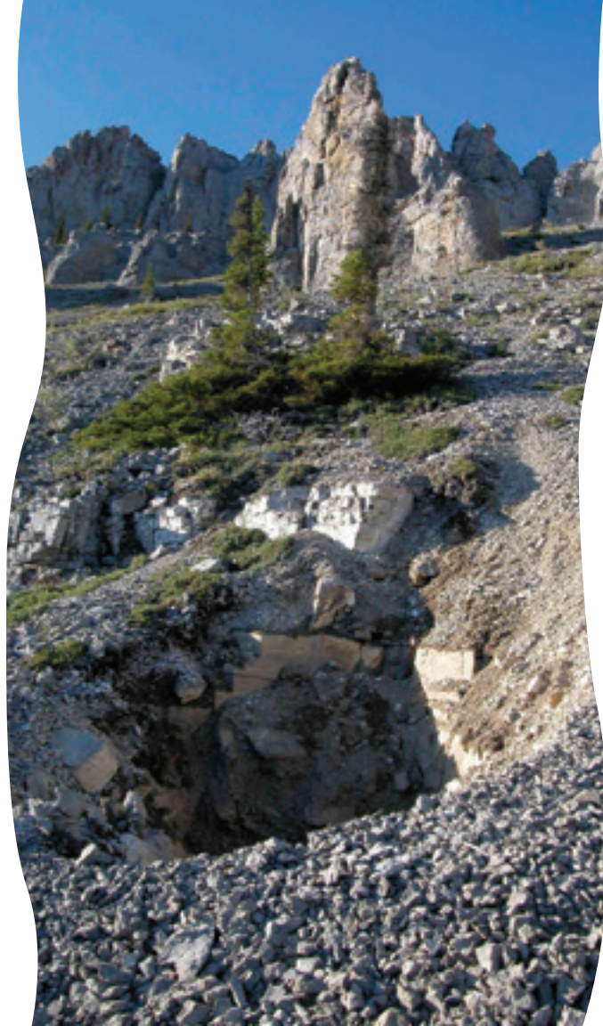
Collapse on the slopes of Chii Ch'á'an Ddhàa
