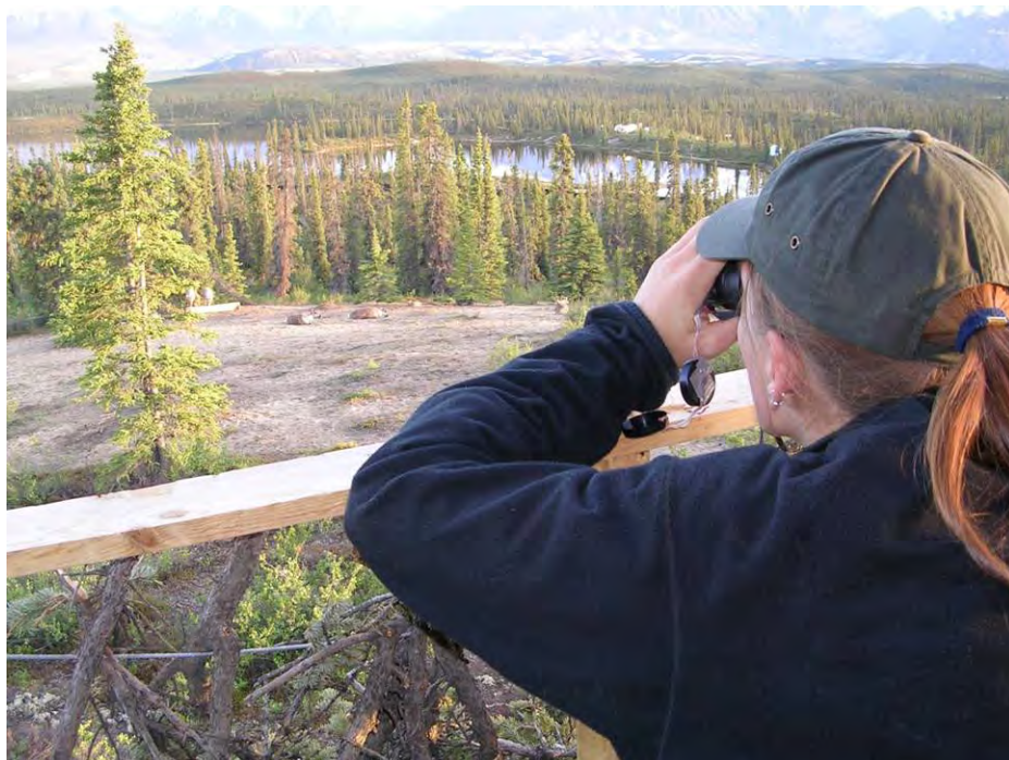
Plate 5. Top photo: Nathan Ferguson (left) and Lorne Larocque constructing a tree-top observation platform (blind) within the enclosure at Boundary Lake, April 2004. Bottom photo: Sara Nielsen keeps a careful eye on caribou in the pen in May 2005.
