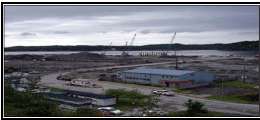
Current perspective of Fairview Terminal & construction (Sep 2006)
