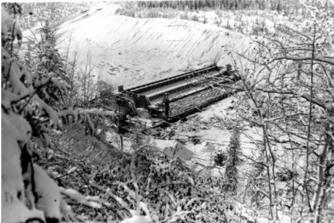
Mayo Hydro Project, the storage dam under construction, October 1952. David R. Duguid Collection
