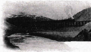
THE TRESTLE THROUGH LEWIS LAKE
