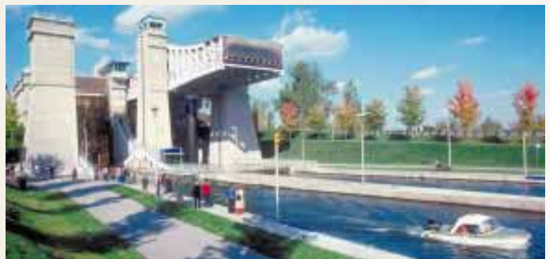
Peterborough Liftlock, Ontario World's Highest Hydraulic Liftlock (1896-1904)
