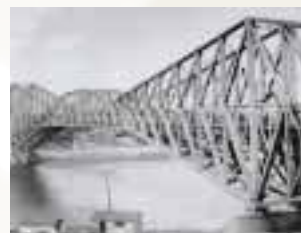
Québec Bridge, Quebec The Longest Clear-Span Cantilever Bridge in the World
