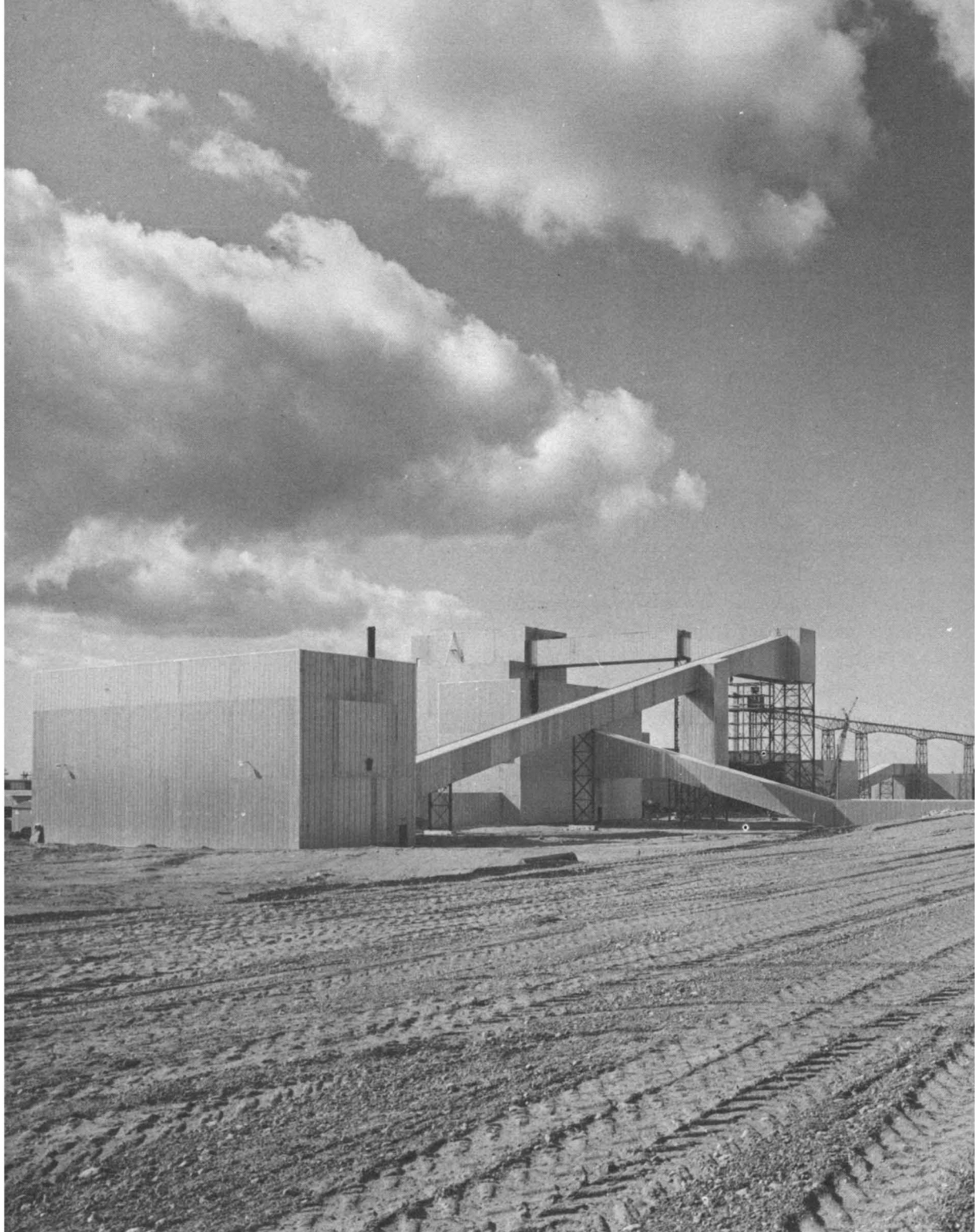
The modern concentrator at Pine Point includes zinc-coated steel siding for protection against corrosion and severe winter weather.
