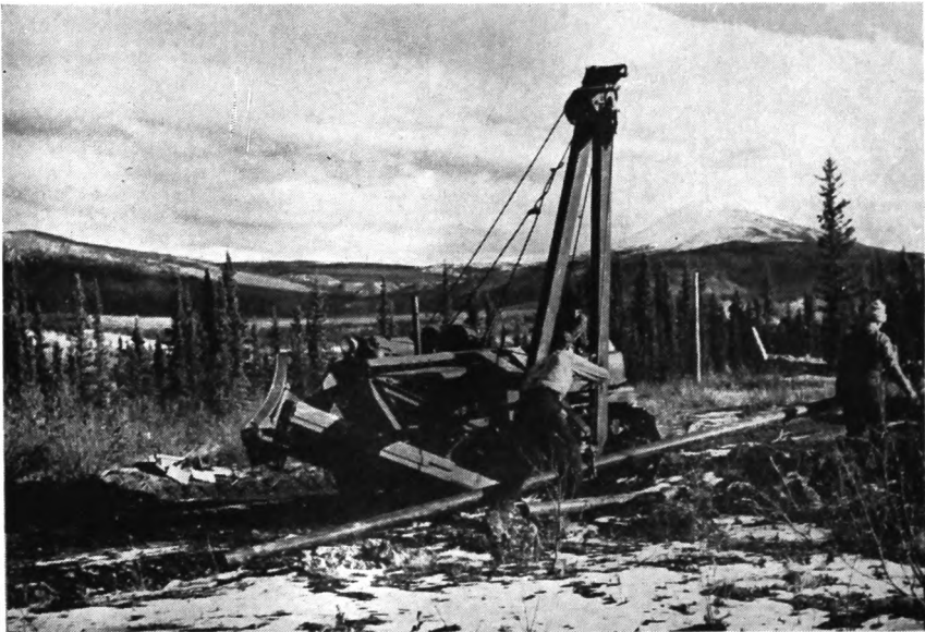
But the pipeline forged ahead.
