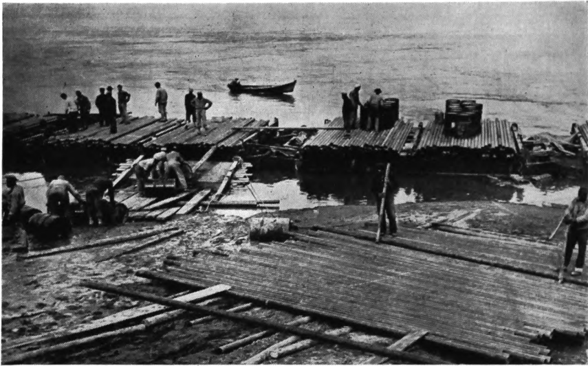
8,000 tons of pipe had been brought down river on ponton rafts as far as Great Slave.
