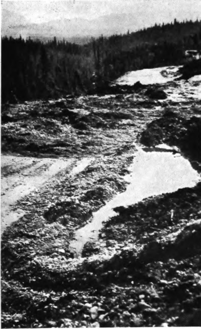
Mushy sidehills slid down over the new road.
