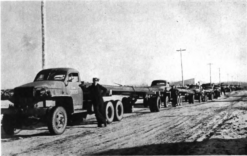
Each truck is carrying half a mile of pipe. With the completion of the Alaska Highway, freight moved smoothly to Whitehorse.
