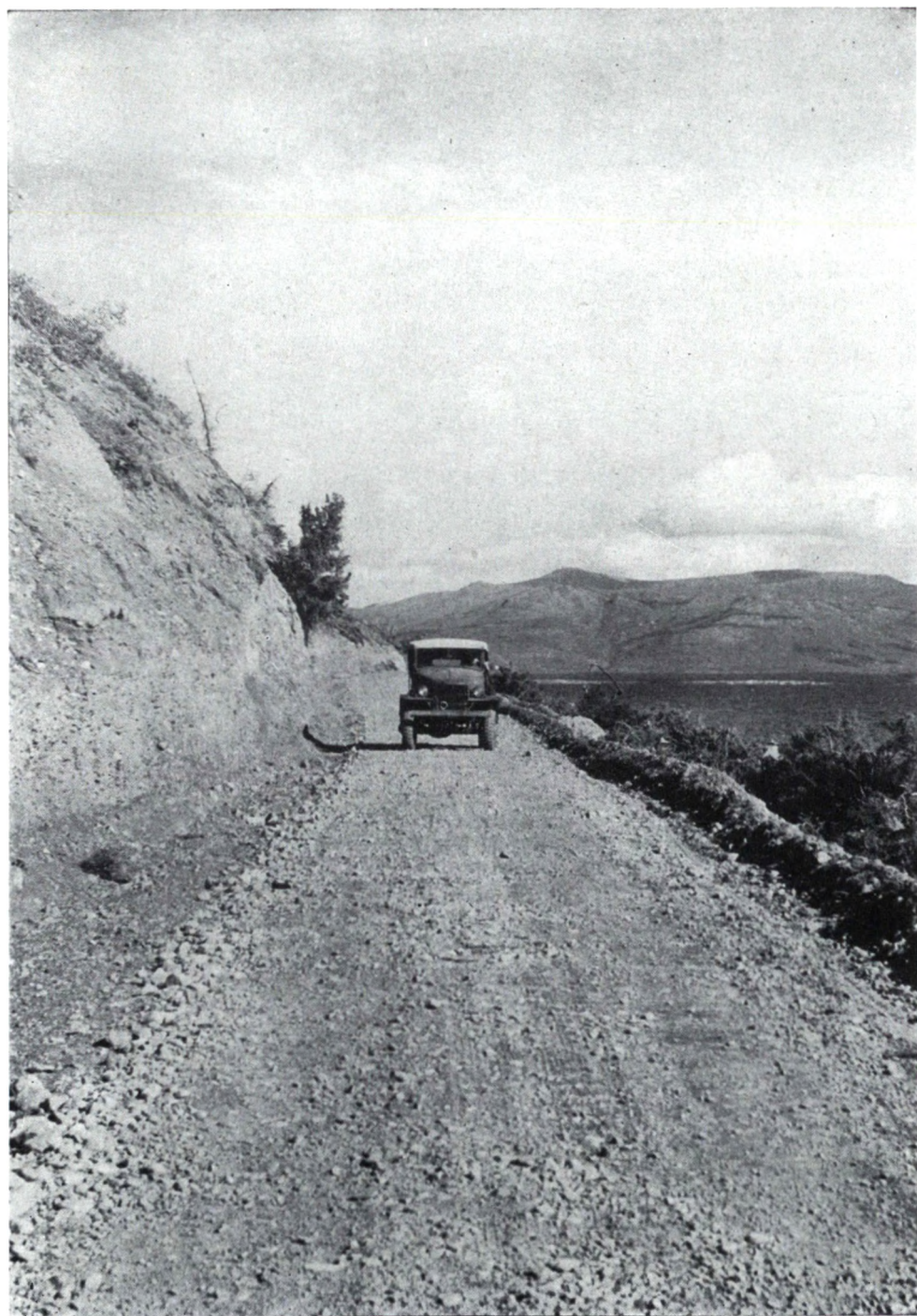
CUT ALONG MOUNTAIN BASE
