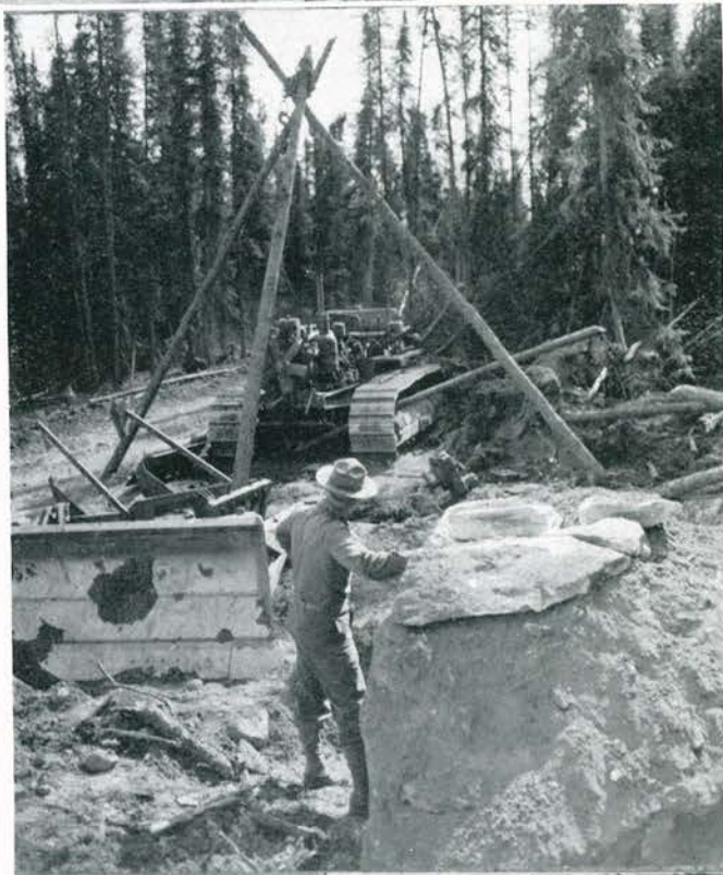
Block and tackle swung from a log shears demonstrate the 340th's methods of repairing heavy equipment in the field.
