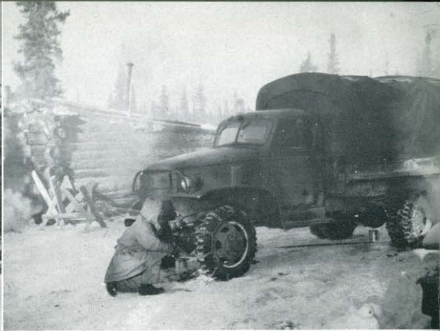
In the dead of winter, trucks were exceedingly difficult to start. This driver has built fires under the differentials—a standard practice necessitated by temperatures ranging down to 70 below zero.
