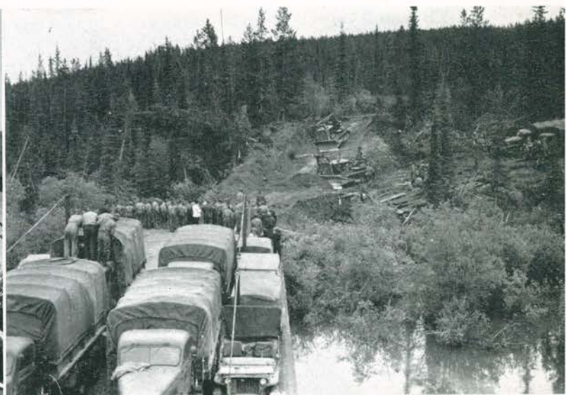
End of the march—Johnson's Crossing. Two D-8 cats with dozer blades working on the fill for Johnson's Landing, Teslin Lake.
