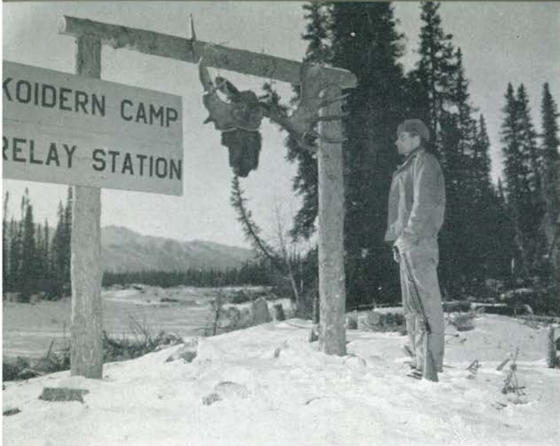
Relay stations, such as this one at Koidern, were established by the 340th for Fairbanks Freight maintenance. Drivers were changed at every station.
