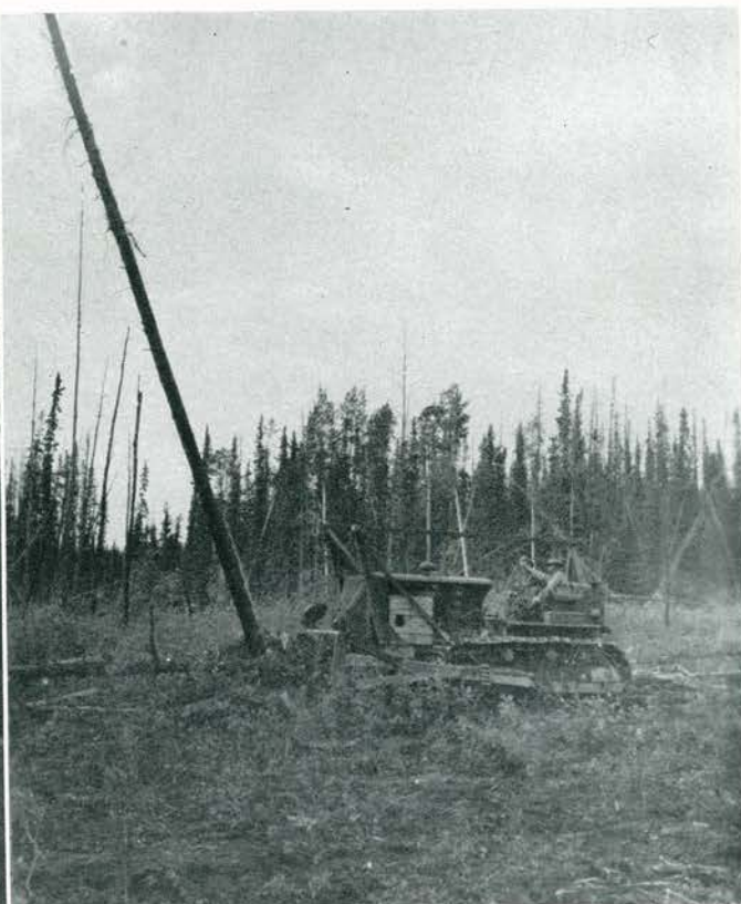
Trees, large or small, topple and are shoved aside to make way for the Alcan Highway.
