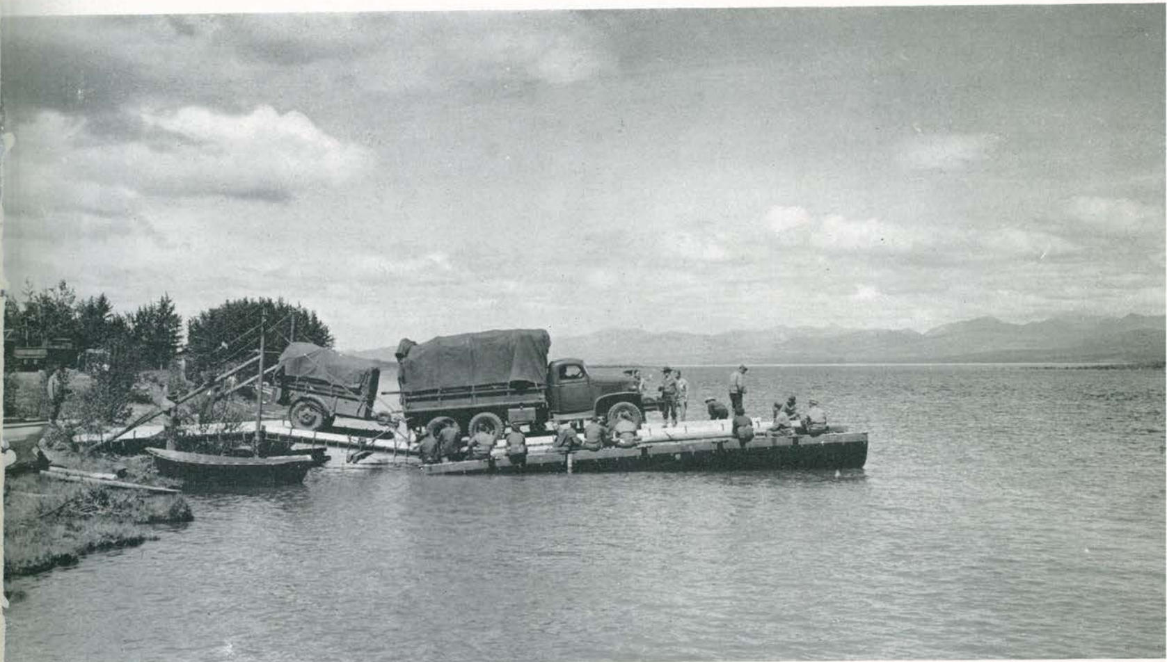
Welcome break in the cross-country hike came at the Tagish river. Here a truck and trailer are being loaded on a ferry by the 73rd Ponton Company platoon attached to the 340th.
