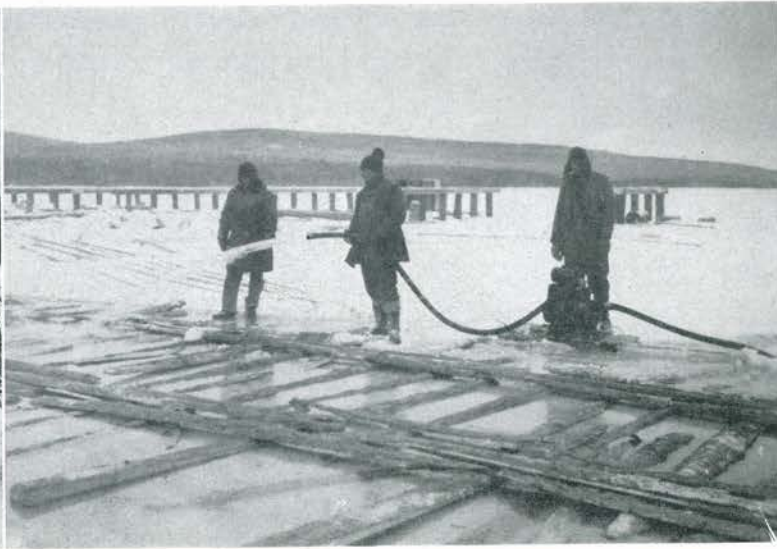
Strengthening the Nisutlin ice crossing by pumping water to freeze over a base of slabs.
