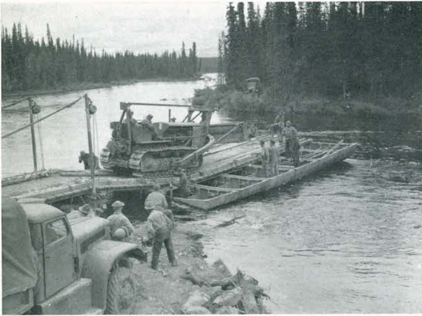
The 73rd Ponton Company platoon, attached to the 340th, played an important role at each stream crossing. Here a D-8 "cat" is being loaded on the ponton ferry at Morley River.
