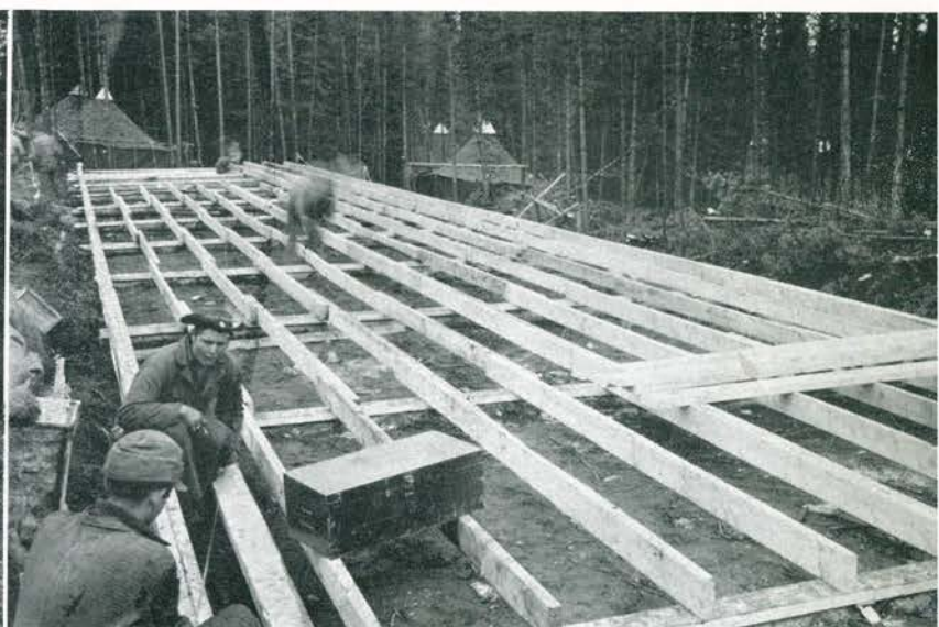
Stringers are being laid for a mess hall at Morris Lake, late in November.
