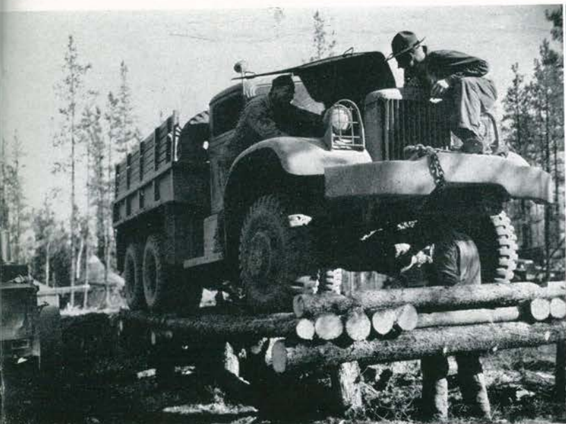
Grease and service rack, courtesy Yukon forest timbers. R.S.O. freight trucks serviced at Watson Lake.
