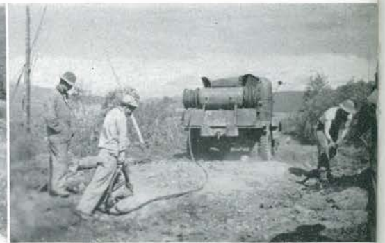
Company F drilling some rock outcropping in preparation for blasting.
