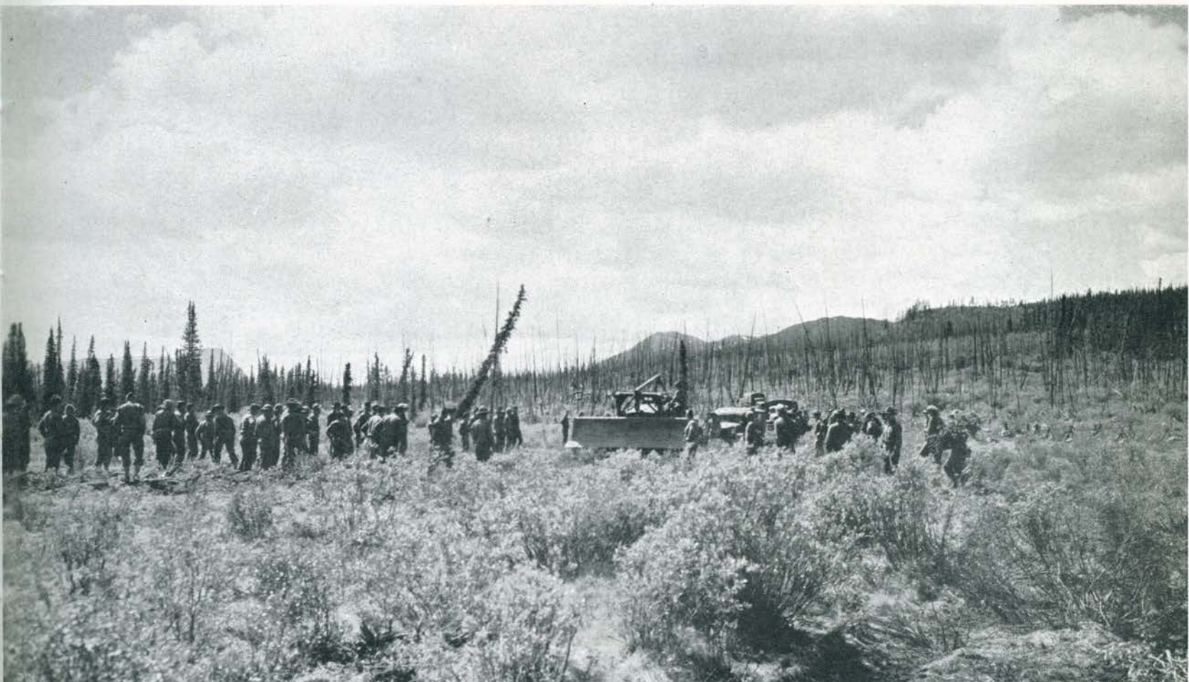
Swamp, deceptively soft and deep, bogs the ration trucks accompanying the expedition. Arms and packs are stacked while the men lay a bit of rough corduroy.
