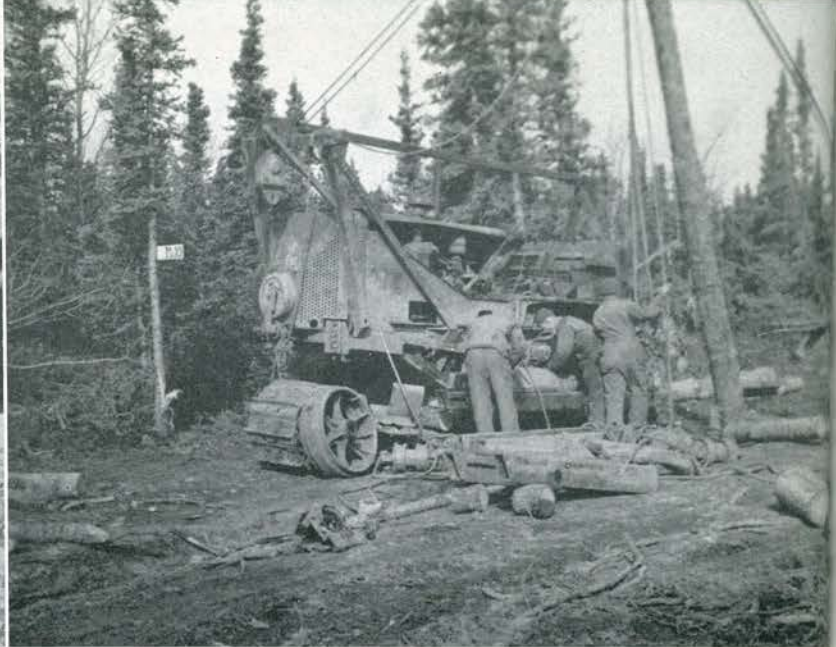
Company F engaged in a major repair job. Equipment used the previous year by 18th Engineers was hard pressed to last thru another season.
