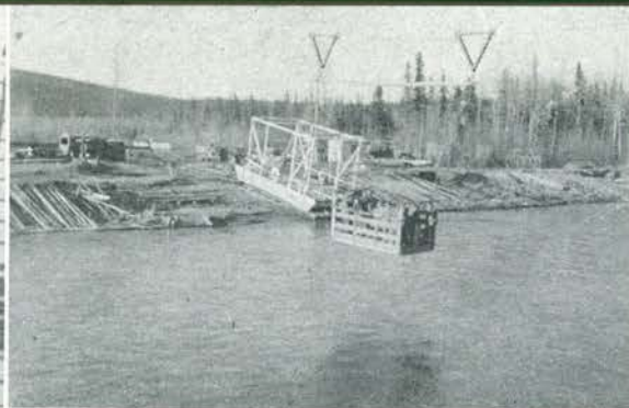
High line rigged up by C Company at the Tanana river.
