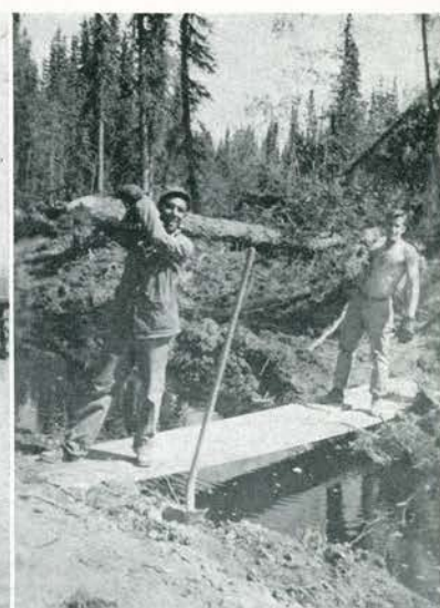
Two C Company stalwarts carry timber for work below Snag Creek.
