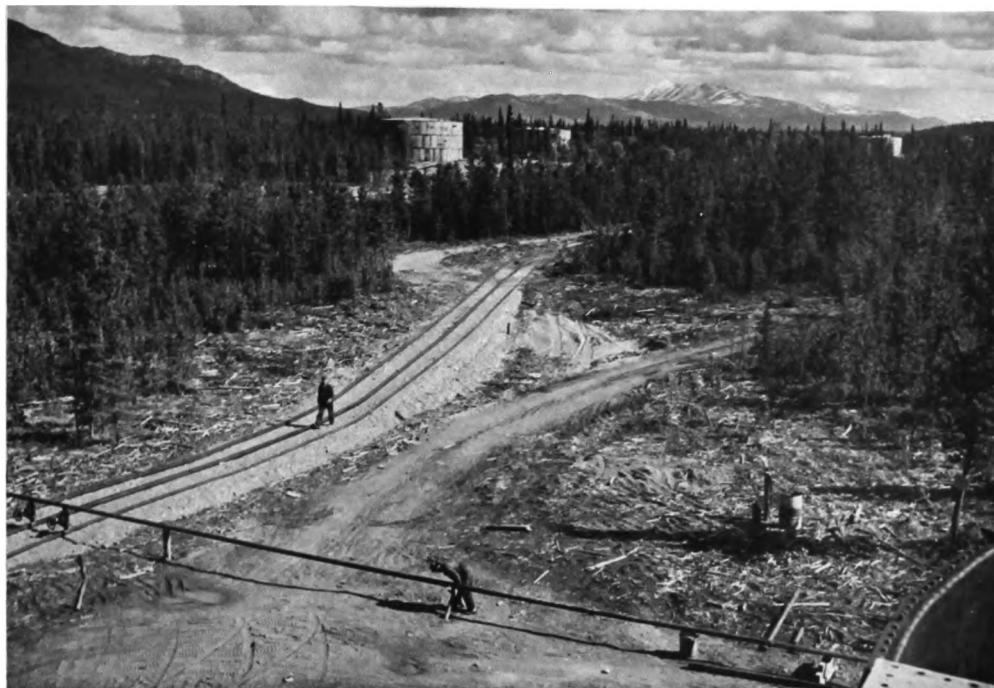
FIG. 13—Tank farm at the Whitehorse end of the pipe line. (National Film Board.)
