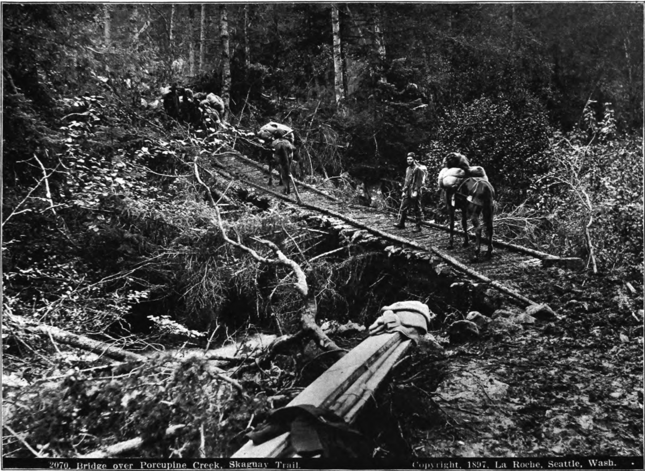
2070. Bridge over Porcupine Creek, Skaguay Trail.
