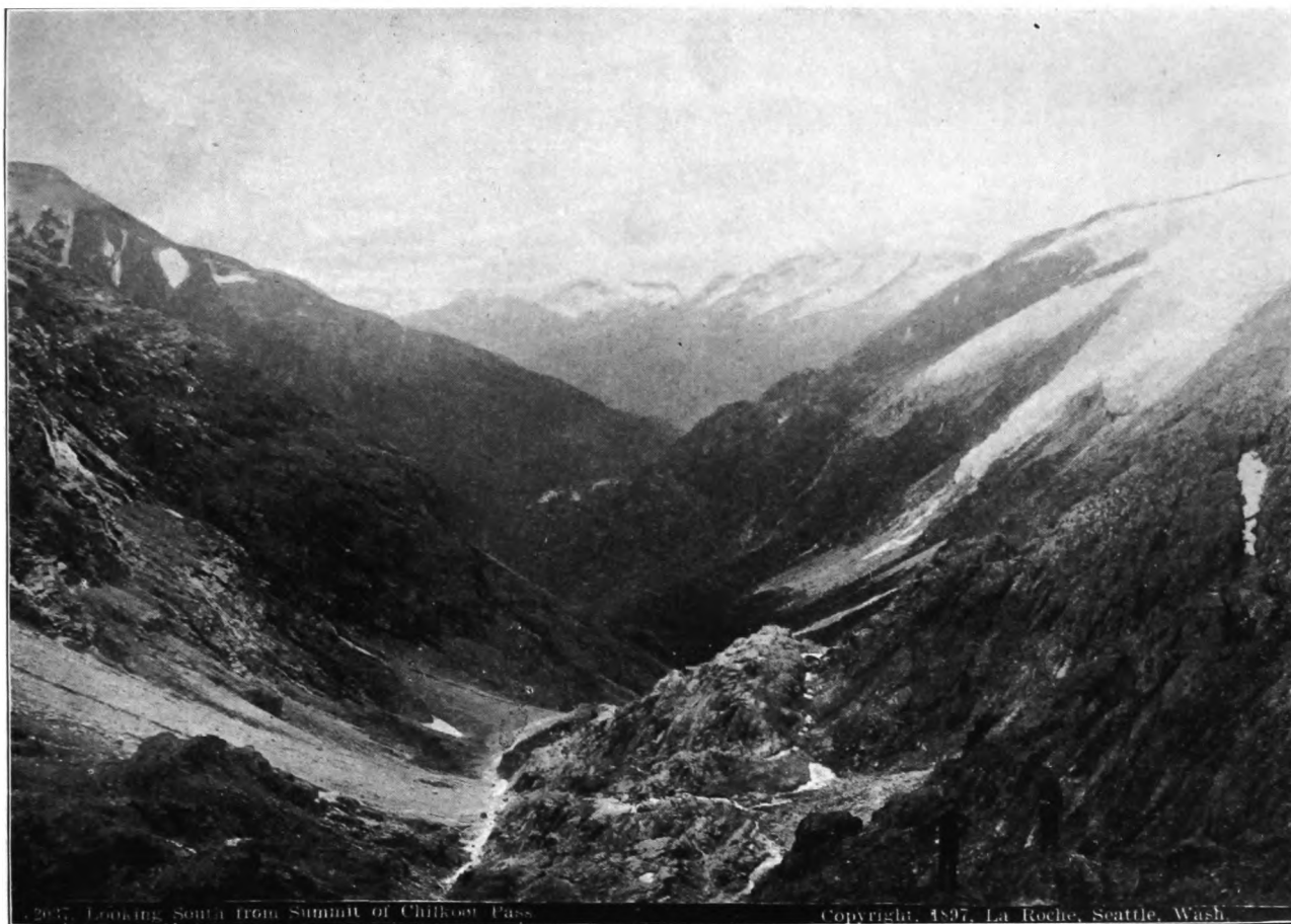
LOOKING SOUTH FROM SUMMIT OF CHILKOOT PASS. —A magnificent panorama of a route traversed for the last seventy-five years by the Indians and during the past summer by at least 4,000 goldseekers. It was the glacier on the right that broke, destroying a number of tents on the Sheep Camp, in September. (2037.)
