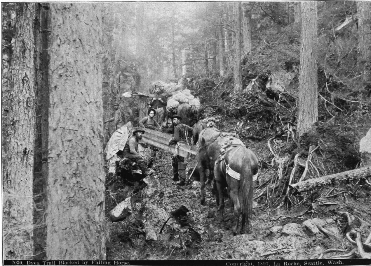
2030. Dyea Trail Blocked by Falling Horse.
