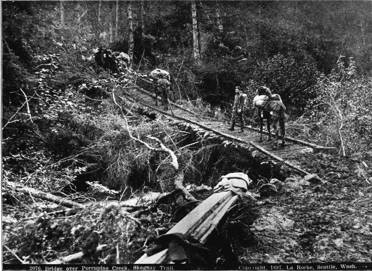
2070. Bridge over Porcupine Creek, Skaguay Trail.
