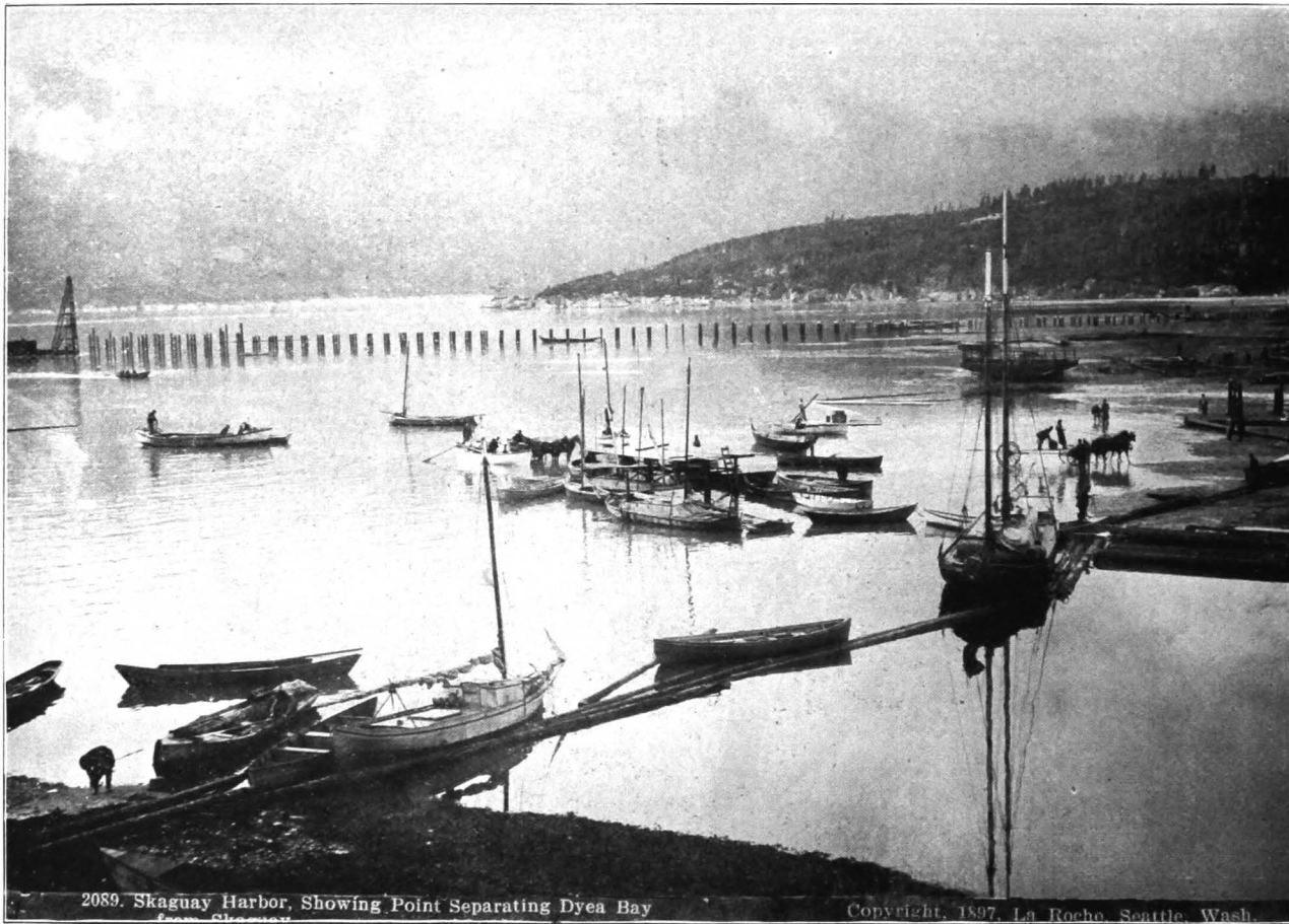
2089. SKAGUAY HARBOR, SHOWING POINT OF LAND SEPARATING DYEA BAY FROM SKAGUAY.—This photo was taken September 12, 1897, at high tide, showing piles driven for one of the three wharfs that were in course of construction; also showing boats used in bringing passengers and outfits from the steamers to the shore, and for transporting from Skaguay to Dyea, around the point of land seen in the center of the picture. Distance from Skaguay to Dyea, five and one-half miles. When the tide is out the boats and scows are left high and dry on the beach, and wagons are driven to the boats, and outfits unloaded and taken on the wagons up the trail to Ragtown, three and one-half miles,
