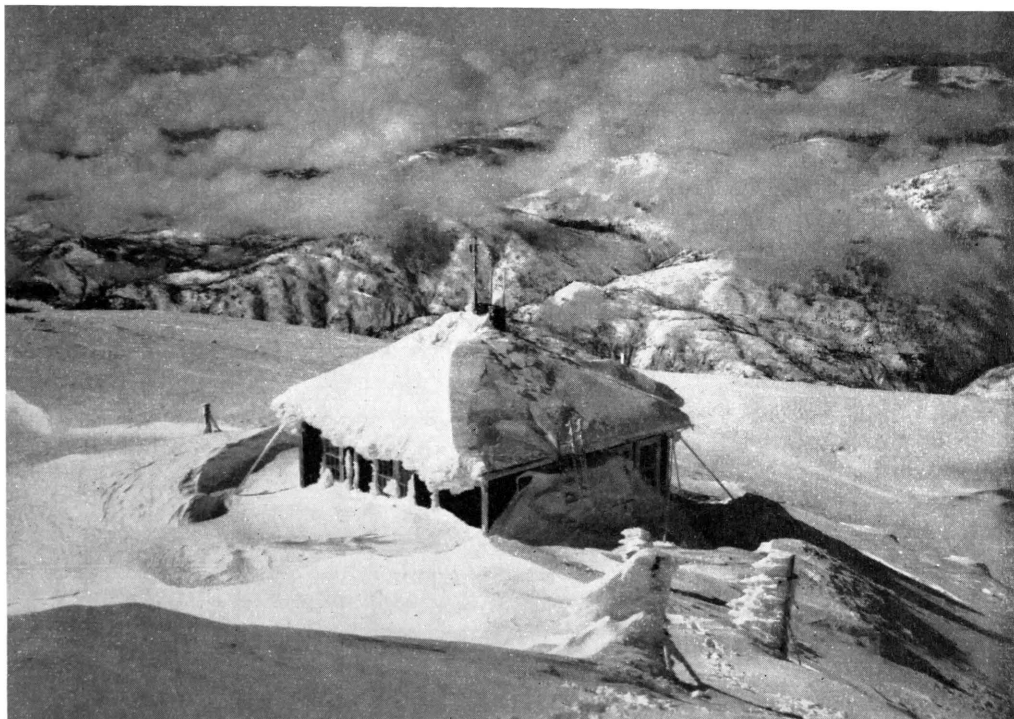
Old Glory Mountain, the highest meteorological station in Canada, altitude 7,700 feet.
